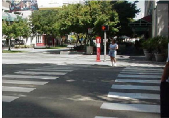
INSTALL LADDER STRIPING WITH 2' WIDE AND 4' LONG WHITE LINES WITH A 4' SPACE AND A 2' WIDE SPACE BETWEEN THE LINES
