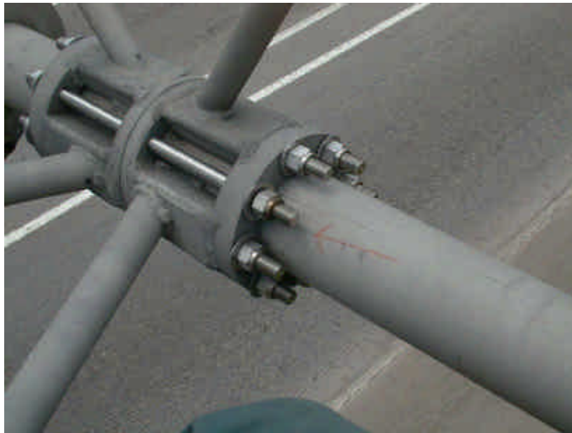
Figure 4c.2 Connection – In Line Chord, ATL Type Sign Support (Alternate) Condition State – Fair: 1 out of 8 (12.5%) bolts loose.
