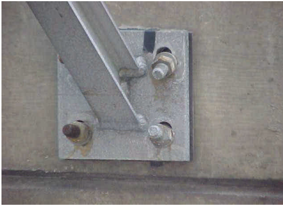
Figure 4a.3 Connection - Base, Attachment of Bridge Mounted Sign Support to Fascia
