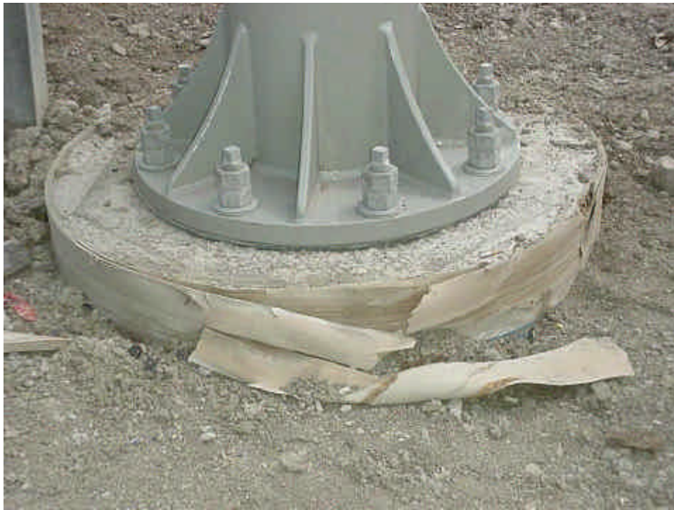
Figure 1c.3 Foundation - Bearing Surface, Leg with Rubber Pad Condition State – Good: Rubber pad in contact over most of the area.
