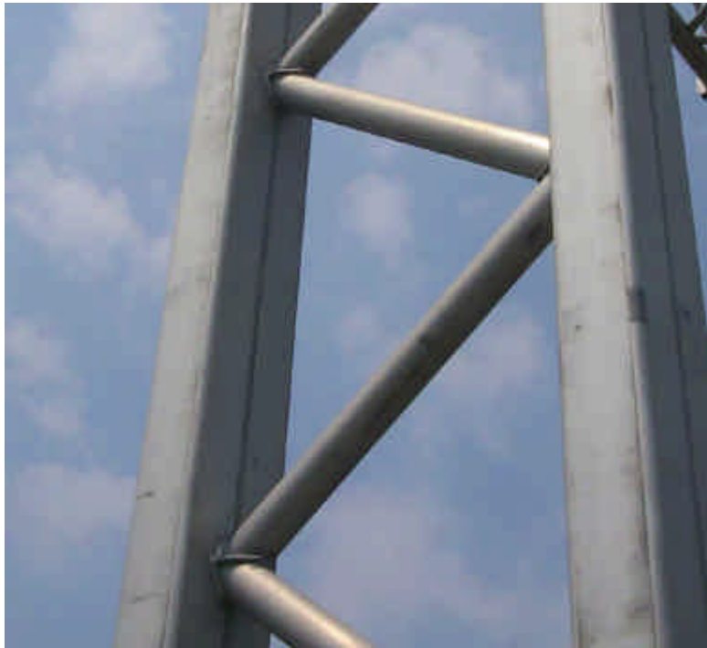
Figure 2b.3 Chords - Leg, ARL Sign Support Condition State – Excellent: No defects. Note: check diagonals for drain holes, possible rehab. need (07)
