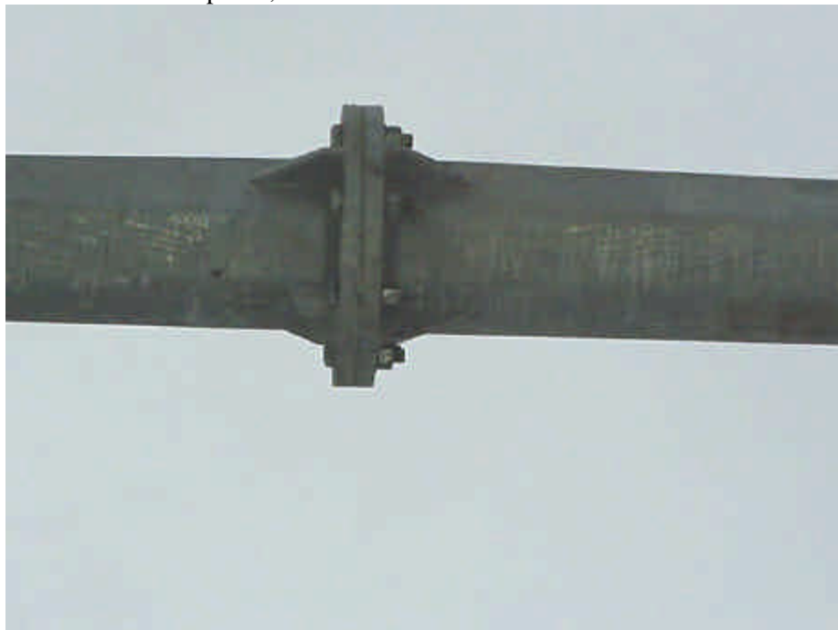
Figure 4c.5 Connection – In Line Chord, Mono-Tube Sign Support Condition State – Good: All bolts tight, minor corrosion of plates with no section loss.
