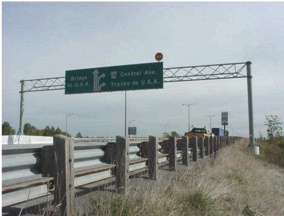
Figure 0.5 Tri-Chord Sign Support (TC)
