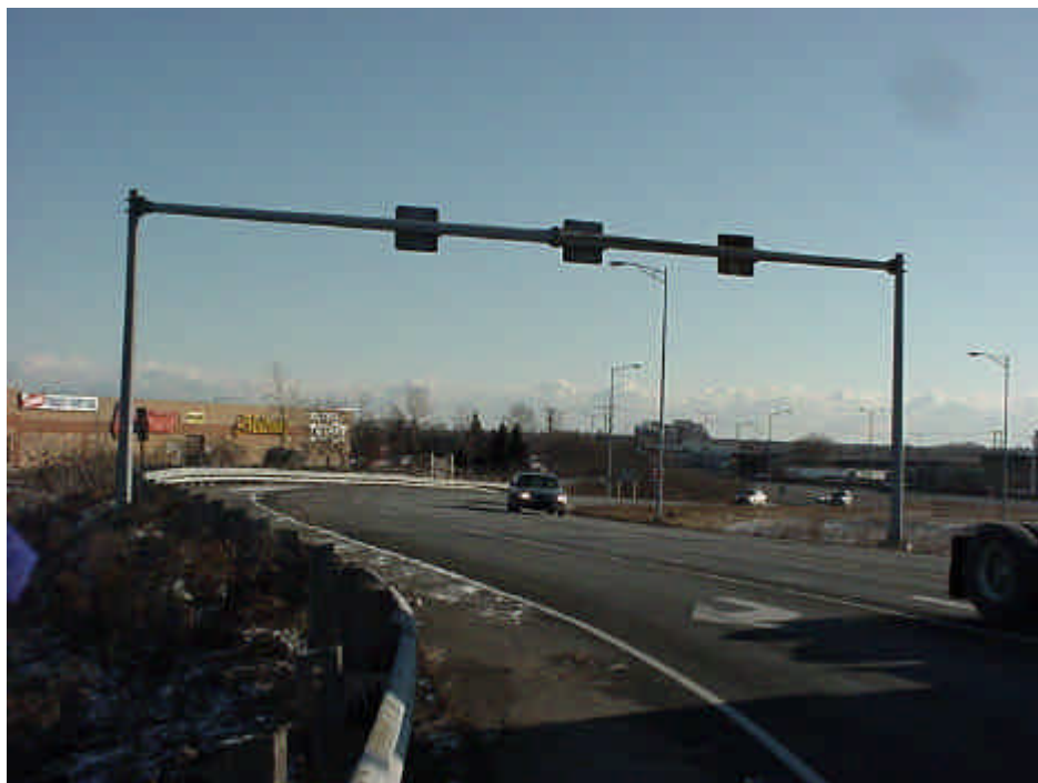
Figure 0.7 Mono-Tube Sign Support (MT)
