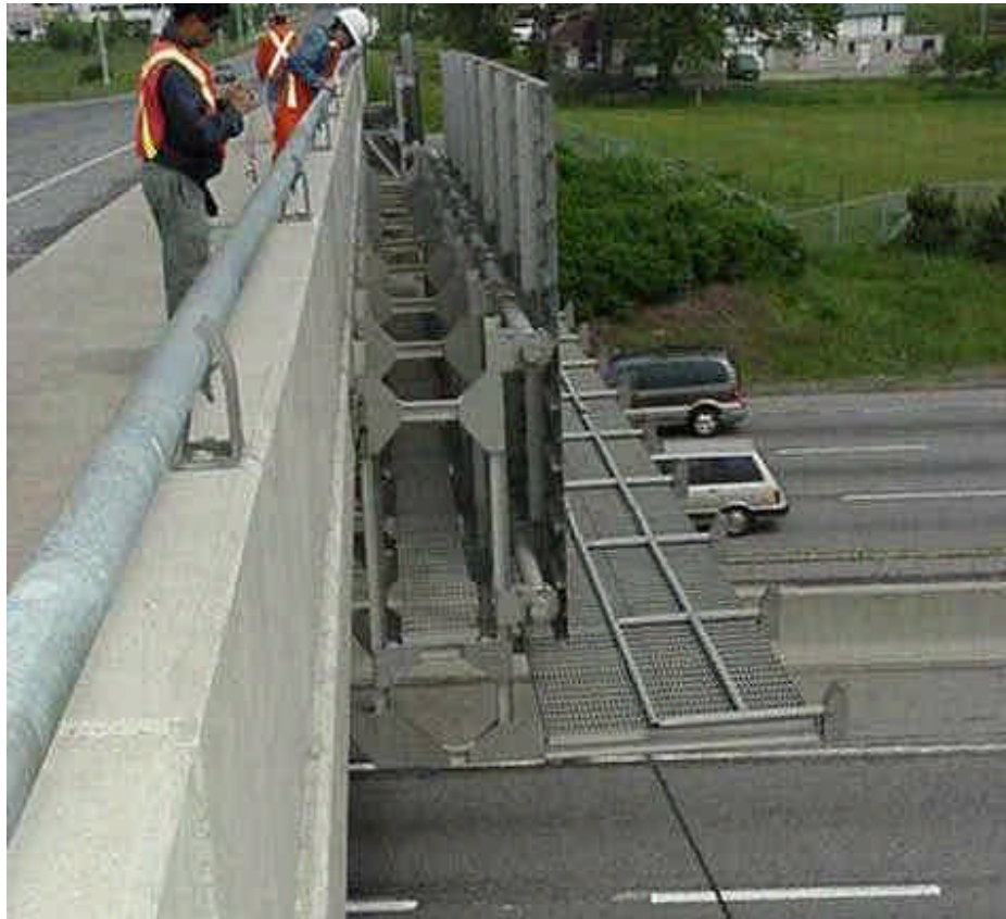
Figure 0.13 Bridge Mounted Sign Support, (BM2S) (Connected at 2 points – soffit and fascia, with walkway and spacer truss behind sign).
