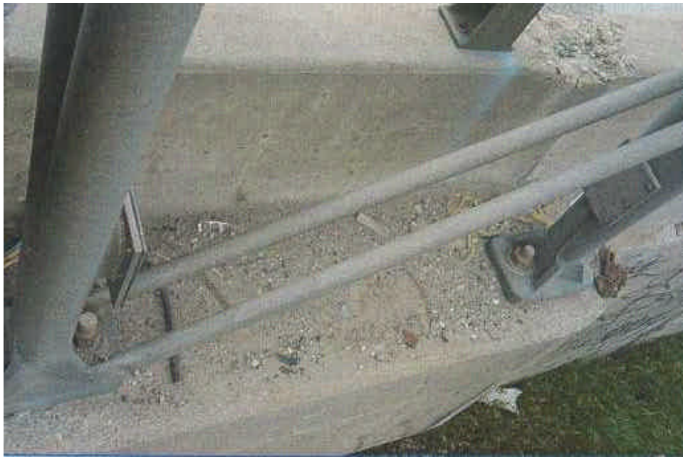
Figure 1a.3 Foundation - Concrete, Bridge Mounted (ATL) Sign Support Condition State – Fair: Medium scaling. Maintenance Need – clean debris (01).
