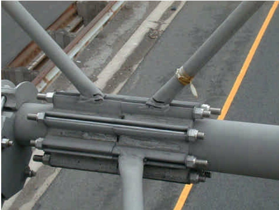
Figure 4c.1 Connection – In Line Chord, ATL Type Sign Support Condition State – Good: Minor corrosion of aluminum casting. Note: Small cracks in the weld of diagonal will not affect chord strength; therefore the cracks are included only with the diagonal element condition rating.
