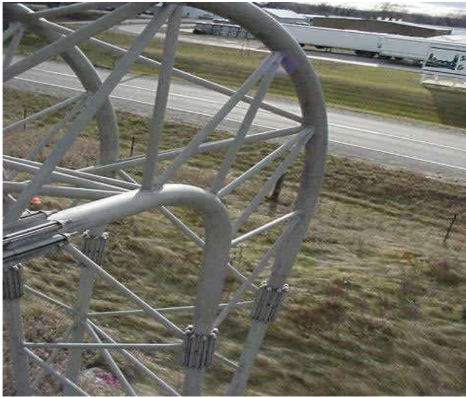
Figure 2c.1 Chords of Corner Arc, ATL Sign Support Condition State – Excellent: No defects.
