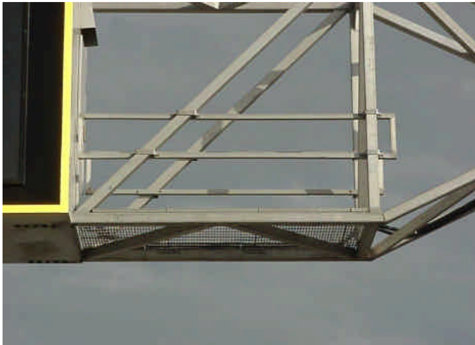
Figure 5f.2 Attachment – Handrail, Attached to CMS-Type Sign Support Condition State – Excellent: Handrail firmly attached and no defects.
