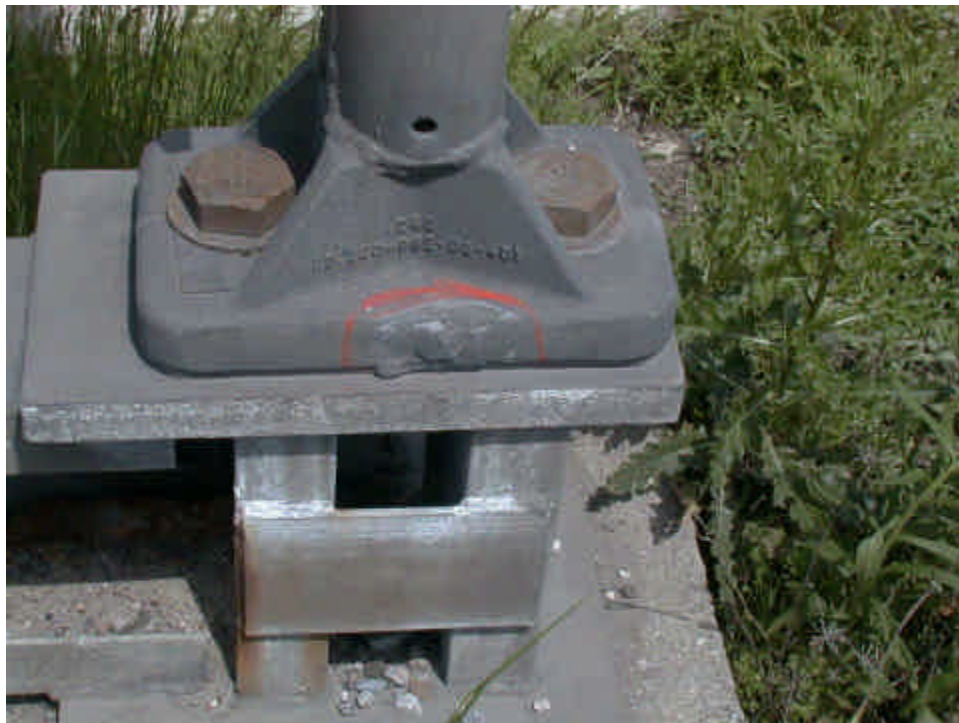
Figure 2a.1 Chord - Base Plate, Aluminum Casting of ATL Sign Support Condition State – Fair: Local corrosion with less than 10% section loss.
