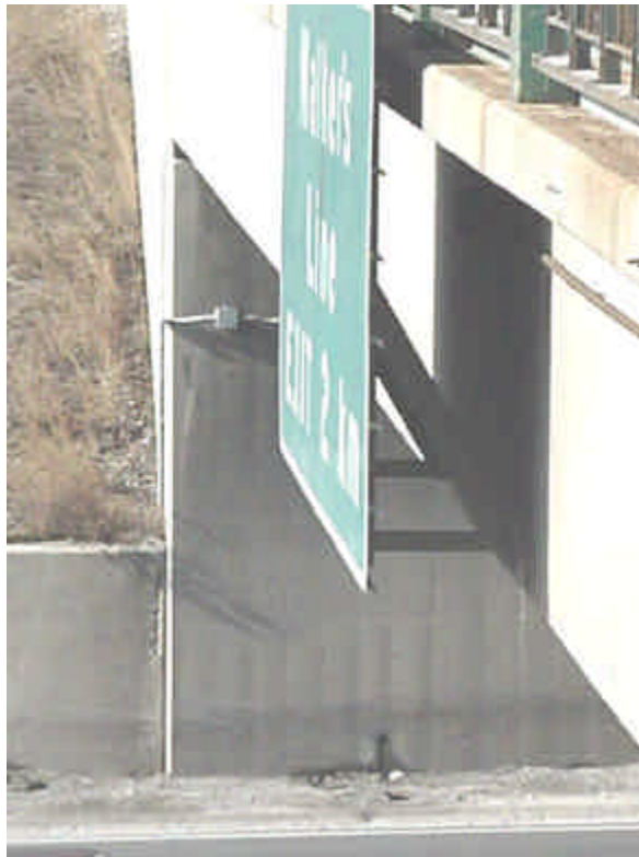
Figure 0.8 Bridge Mounted Sign Support, (BM2) (Connected at 2 points, no walkway)
