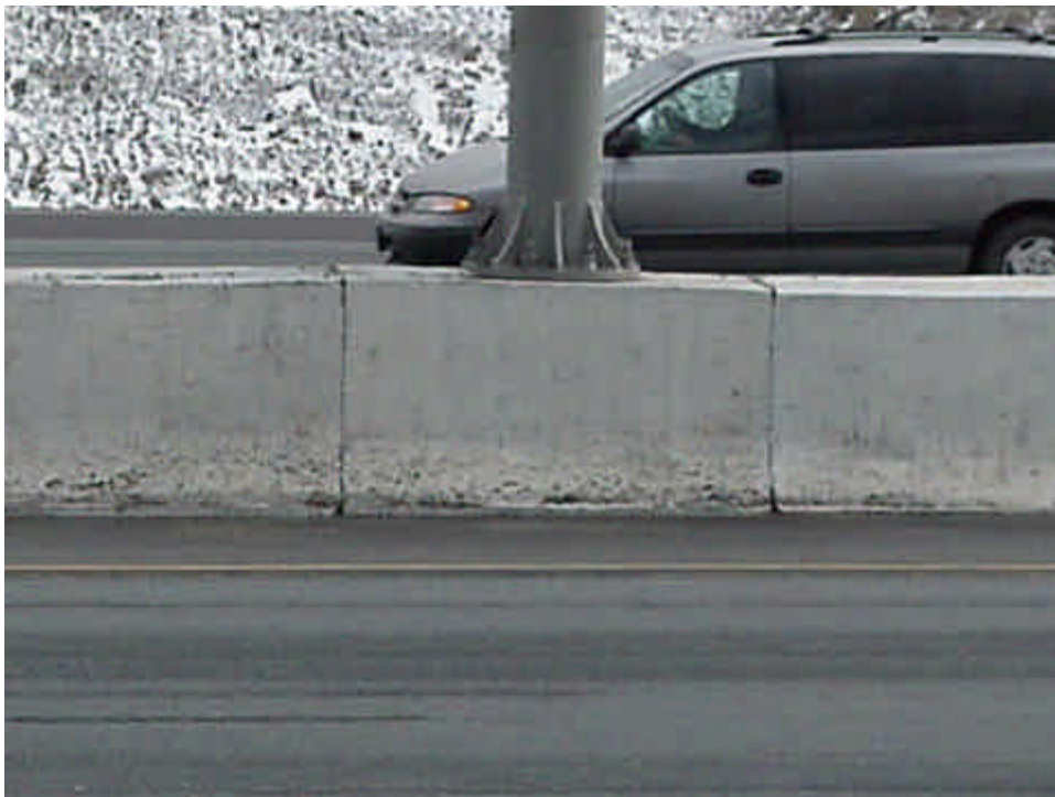
Figure 1a.2 Foundation - Concrete, on Barrier Wall Condition State – Fair: Medium scaling and pop-outs.
