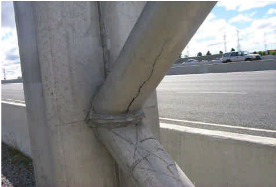
Figure 3a.2 Diagonals – Leg, ARL new Sign Support Condition State – Poor: Underside of diagonal member is cracked. Repair Need – Repair crack in Diagonal (03).
