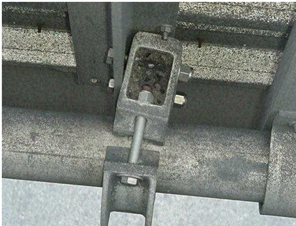
Figure 4d.4 Connection – Sign, Bridge Mounted Sign Support Condition State – Fair: Misaligned cast aluminum clamp.
