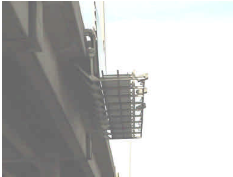
Figure 0.12 Bridge Mounted Sign Support, BM3) (Connected at 3 points – soffit, 2 on fascia, with walkway)
