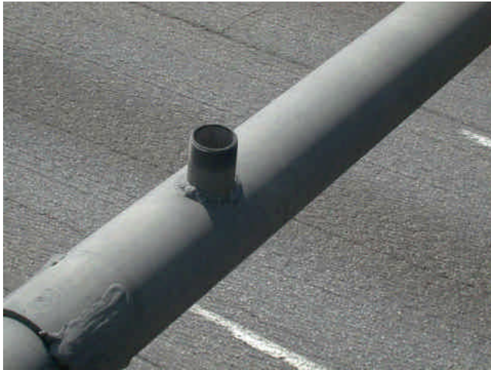
Figure 2d.1 Chords – Horizontal, Aluminum Sign Support Condition State – Good: Note that shop splice is included with chord and not with connection. Minor corrosion with no section loss. Note: replace cover on conduit – maintenance item (04).
