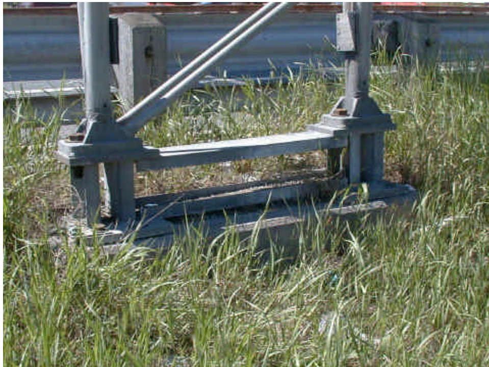
Figure 1b.1 Foundation - Steel Pedestal Under ATL Sign Support Condition State – Good: Light corrosion with no section loss. Maintenance Need – clean debris (01).
