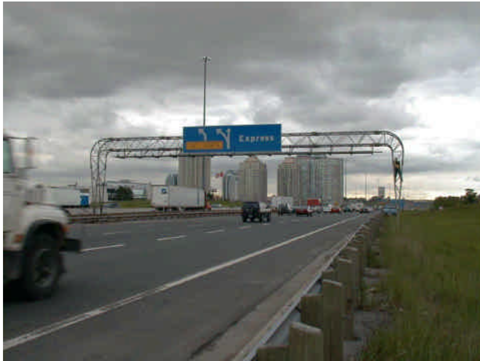
Figure 0.1 Aluminum Tapered Leg Sign Support (ATL)
