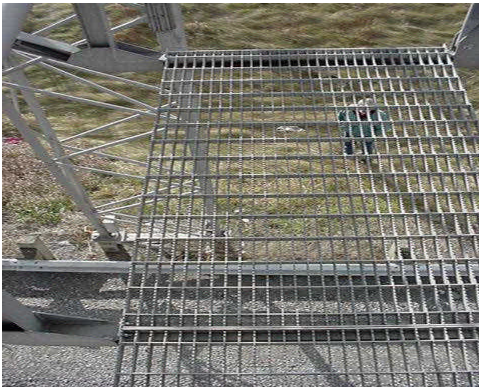
Figure 5e.1 Attachment – Walkway, Attached to Walkway Arms Condition State – Good: Grating firmly attached with minor corrosion and no section loss.
