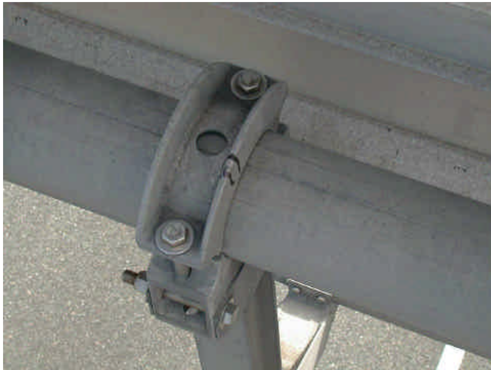
Figure 4f.1 Connection – Walkway Arms, ATL Type Sign Support Condition State – Poor: Crack in aluminum casting. Repair Need – Replace clamp (14).
