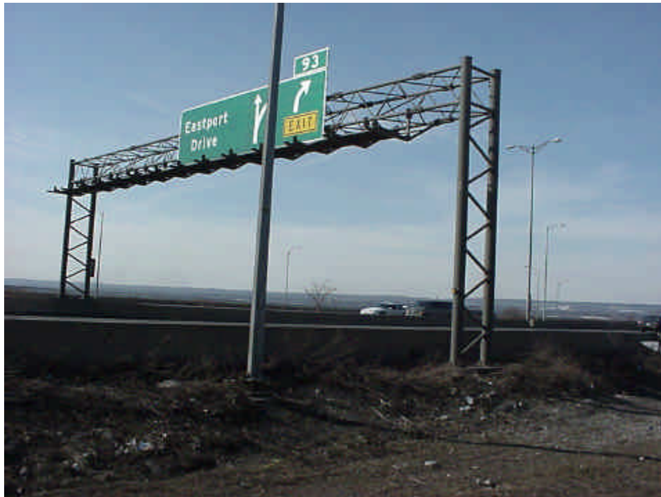
Figure 0.2 Aluminum Circular Leg Sign Support (ACL): Note circular legs
