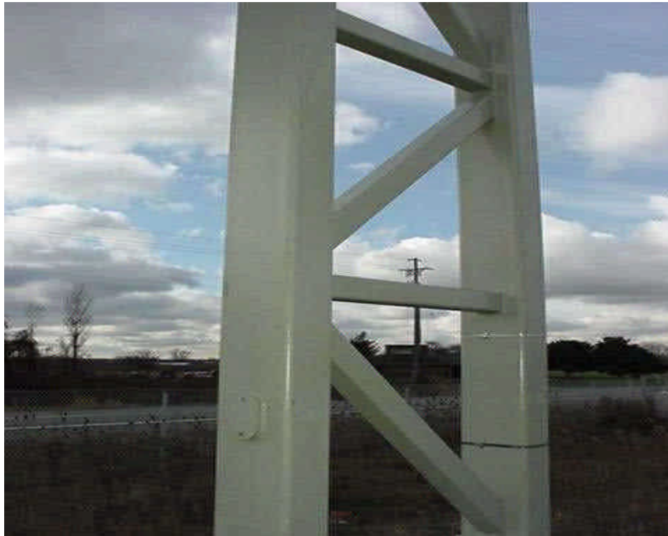
Figure 6a.1 Coating – Chord, Trussed Leg of CMS Type Sign Support Condition State – Excellent: No defects in coating.
