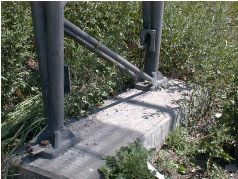
Figure 1a.1 Foundation - Concrete, Projection above ground. Condition State – Good: Minor scaling. Maintenance Need – Clean debris (01) Note: for leg element, cover is missing – maintenance item (04).
