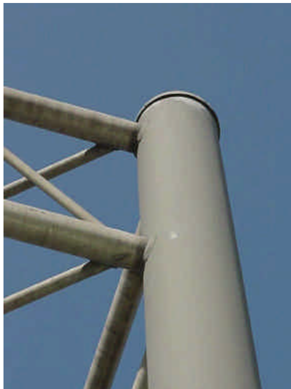
Figure 4b.1 Connection –Leg, ACL Sign Support
