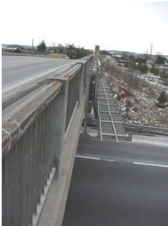
Figure 0.9 Bridge Mounted Sign Support, (BM2) (Connected at 2 points – soffit and fascia, with walkway)
