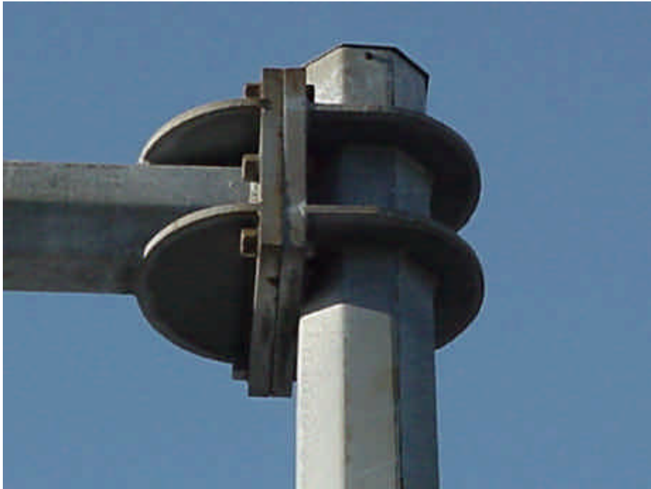
Figure 4b.6 Connection – Leg, Mono-Tube Sign Support Condition State – Good: bolts tight with full contact between plates, minor corrosion with no section loss.
