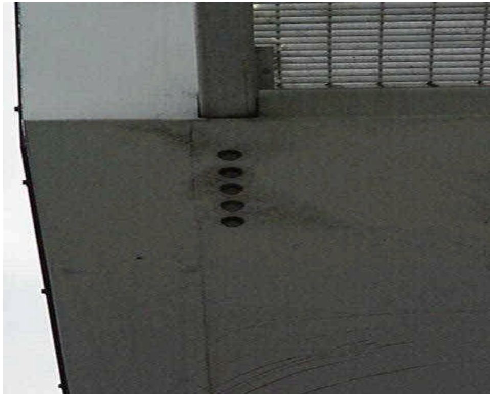
Figure 4c.3 Connection – In Line Chord, CMS Type Sign Support Condition State – Excellent: All bolts in connection are tight.
