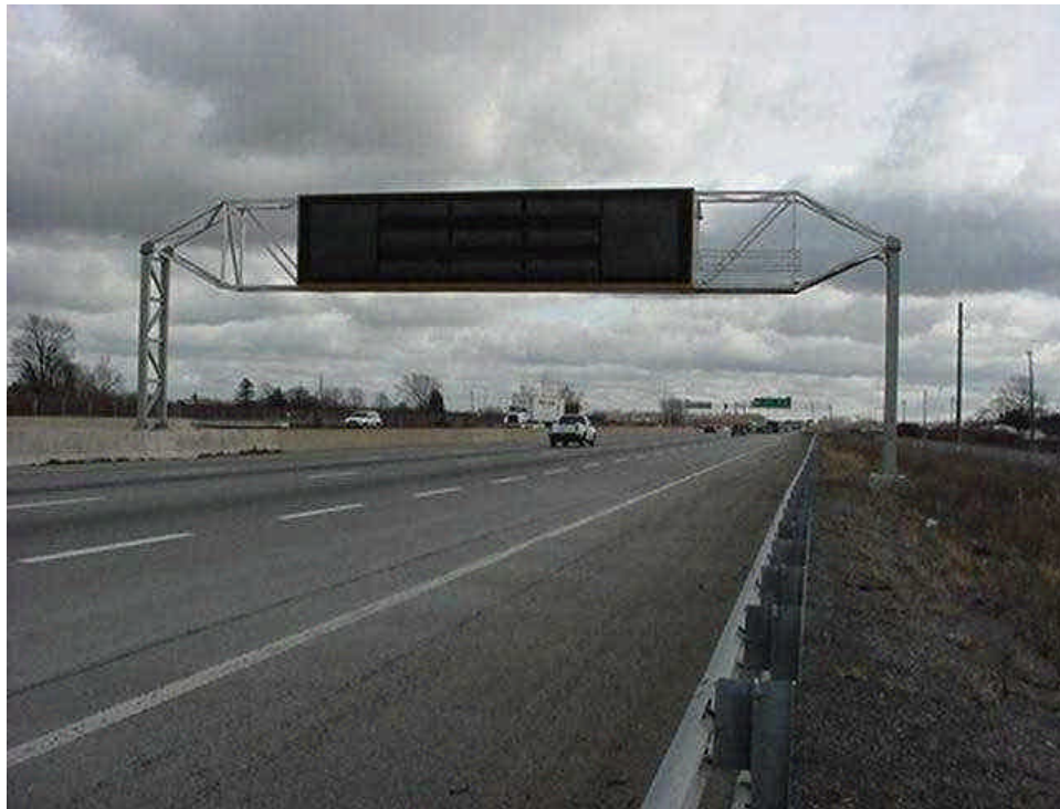
Figure 0.4 Changeable Message Sign Support (CMS)
