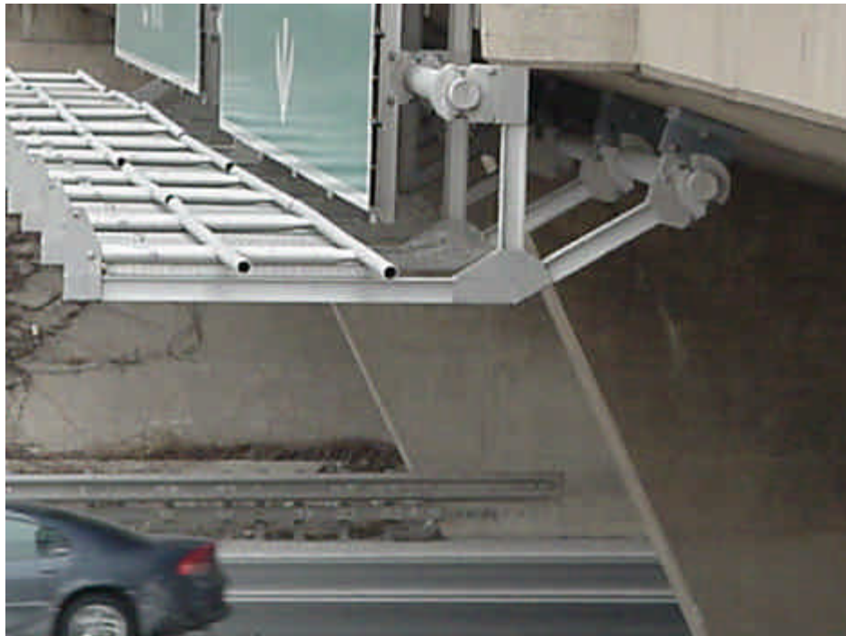
Figure 5d.2 Attachment – Walkway Arms, Attached to Bridge Mounted Sign Support Condition State – Excellent: No defect in aluminum members.
