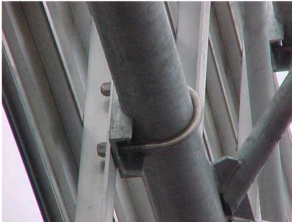
Figure 4d.3 Connection – Sign, Tri-Chord Sign Support Condition State – Fair: Stainless steel U-bolt with no material defects but improper thread projection.
