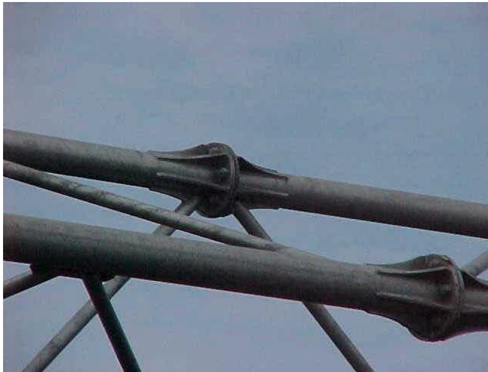
Figure 4c.4 Connection – In Line Chord, Tri-Chord Sign Support Condition State – Good. All bolts are tight with full contact between plates, minor corrosion with no section loss.
