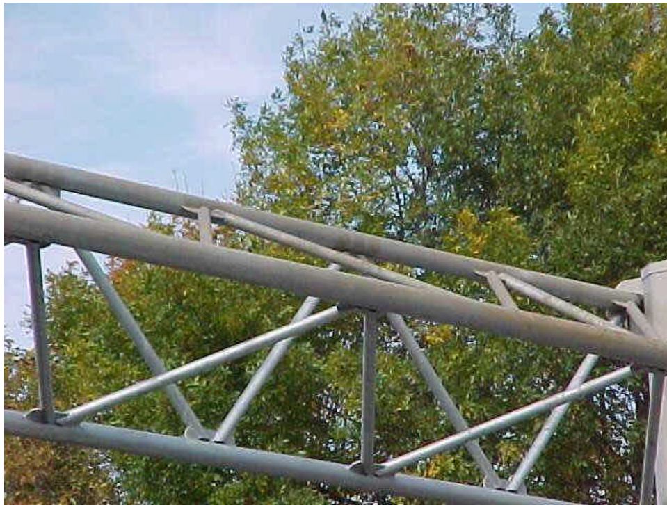
Figure 6a.2 Coating – Chord, Horizontal Truss of Tri-Chord Sign Support Condition State – Fair: Galvanizing wearing off in areas, rust condition rating category 3.
