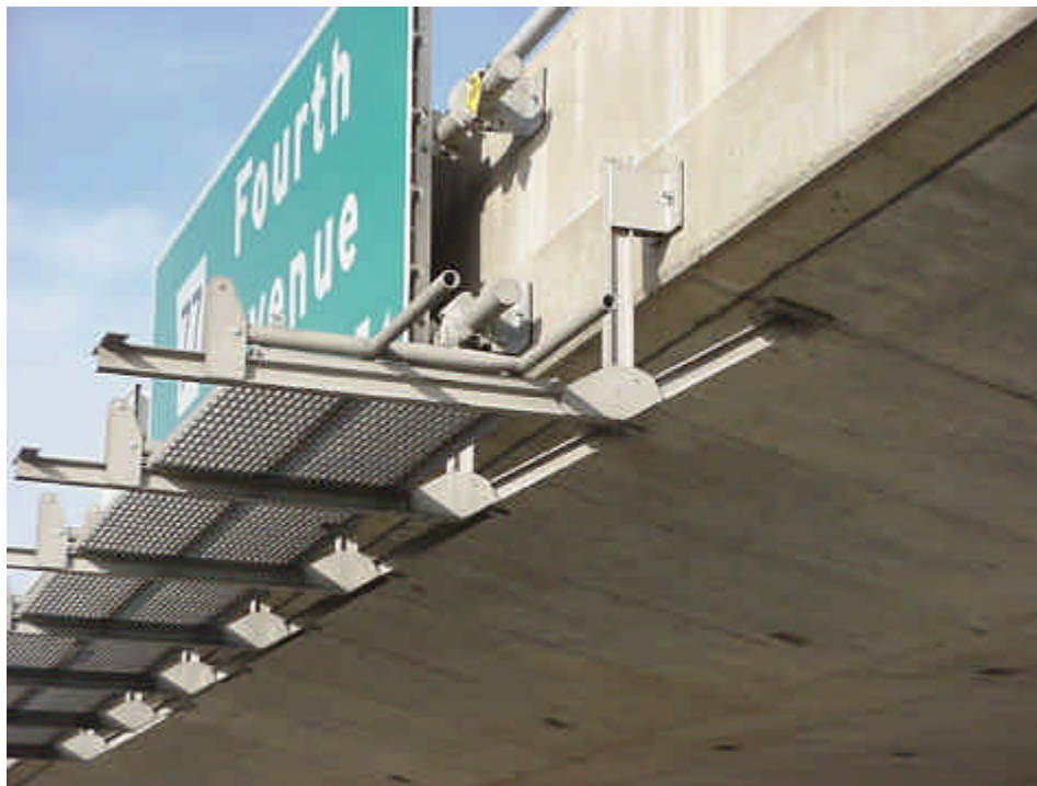
Figure 0.11 Bridge Mounted Sign Support, (BM3) (Connected at 3 points – soffit, fascia and barrier, with walkway)
