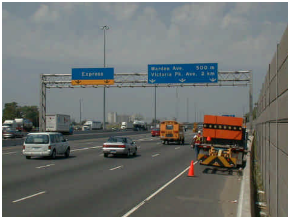
Figure 0.3 Aluminum Rectangular Leg Sign Support (ARL): Note Rectangular Legs.
