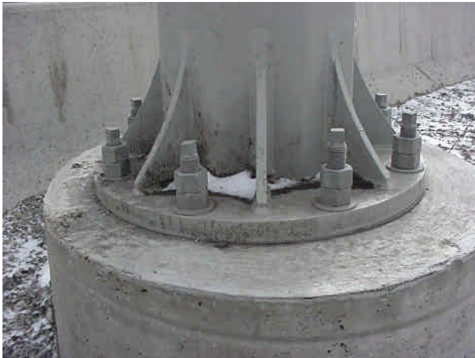
Figure 6c.1 Coating – Connections, Connection at Base of Tri-Chord Sign Support
