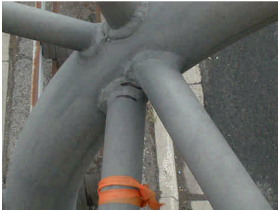
Figure 3b.1 Diagonals – Corner Arc, ATL Sign Support Condition State – Poor: Crack at weld. Repair Need – Repair crack in diagonal at weld (03).
