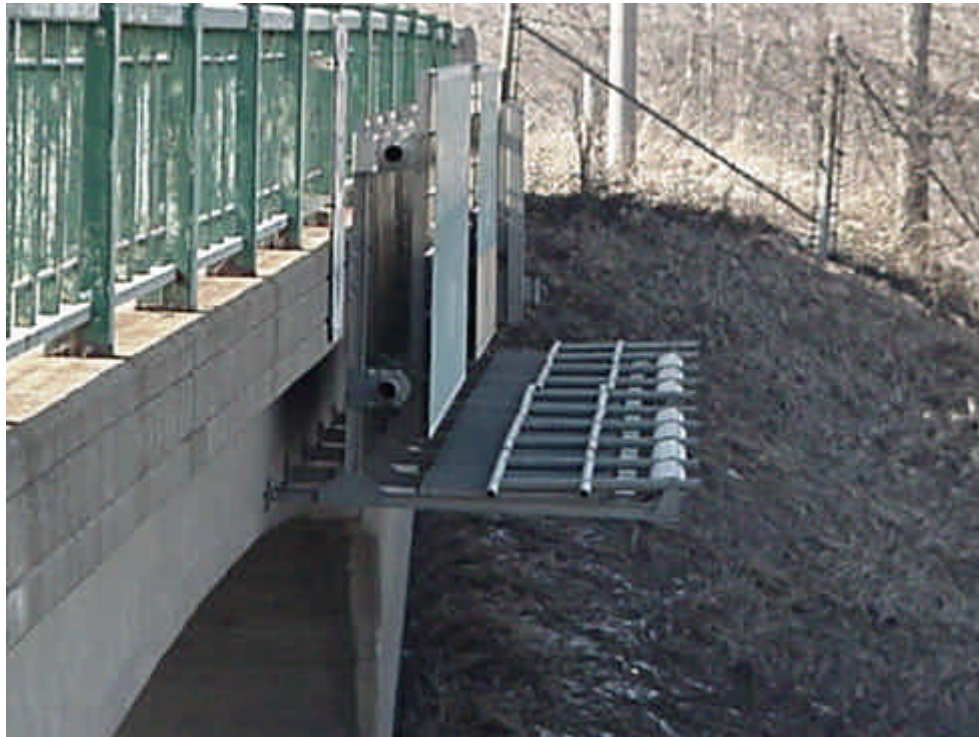
Figure 0.10 Bridge Mounted Sign Support, (BM2) (Connected at 2 points – both on fascia, with walkway)
