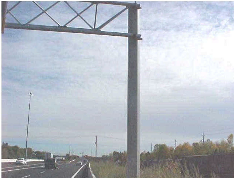
Figure 2b.4 Main Member - Leg, Single Column Leg of Sign Support (TC) Condition State – Excellent: No defects.
