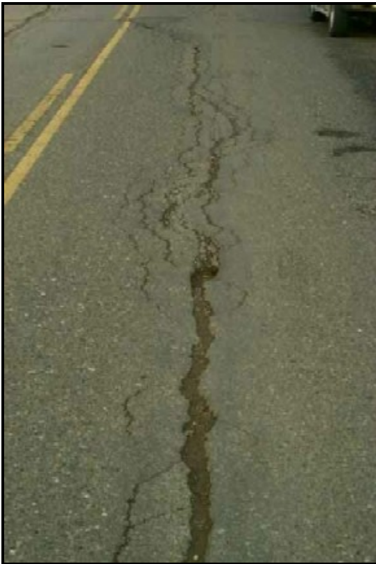
Figure 19 - High Severity MLC (multiple and alligator cracking)
