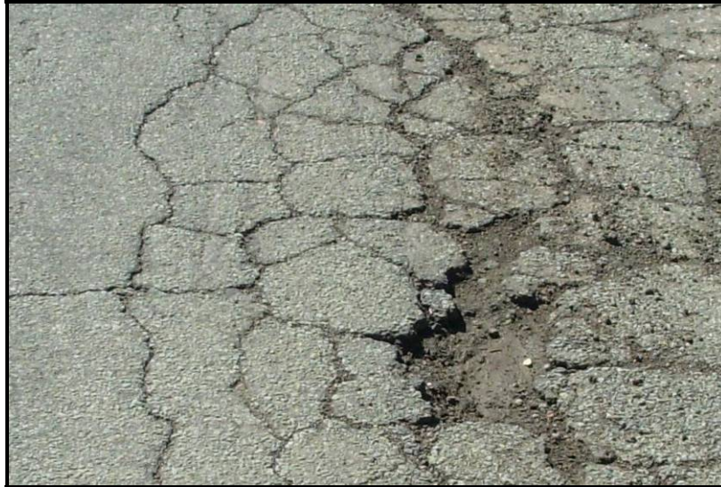
Figure 35 - Low Severity POT (close up view)
