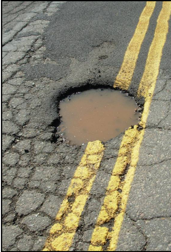
Figure 37 - High Severity Pothole
