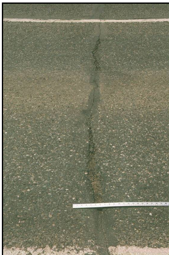
Figure 16 - High Severity TC
