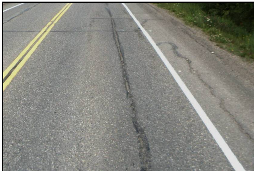
Figure 4 - High Severity LWP
