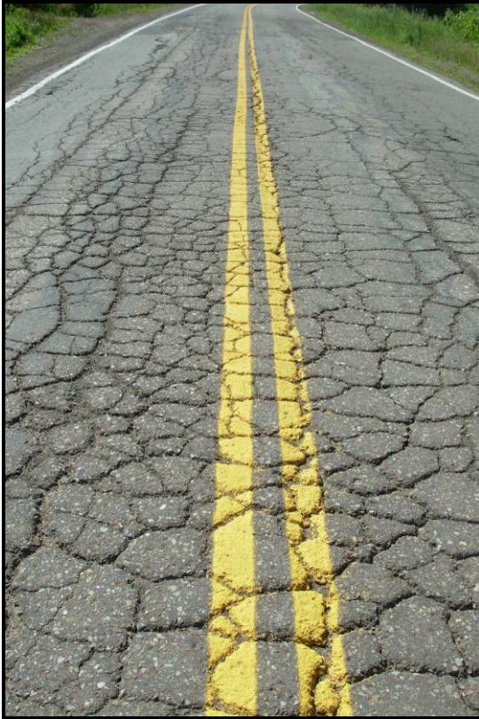
Figure 23 - High Severity AC (spalling and throughout density)
