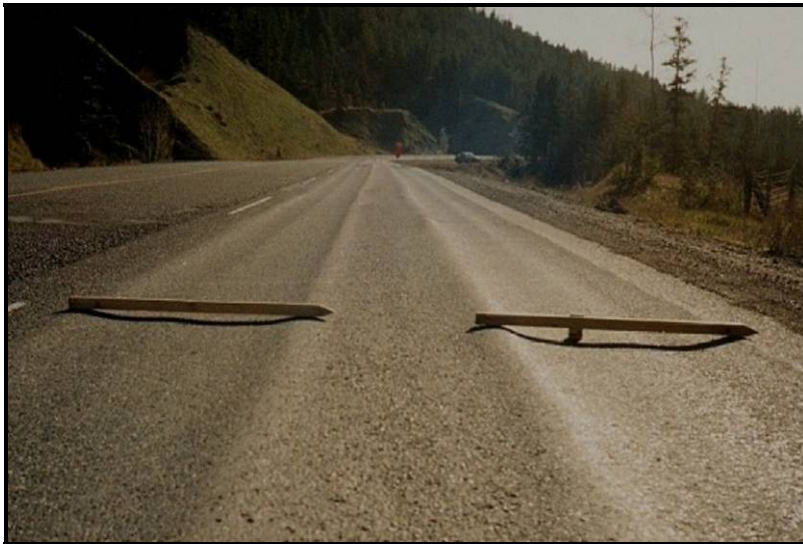
Figure 27 - High Severity RUT with transverse displacement
