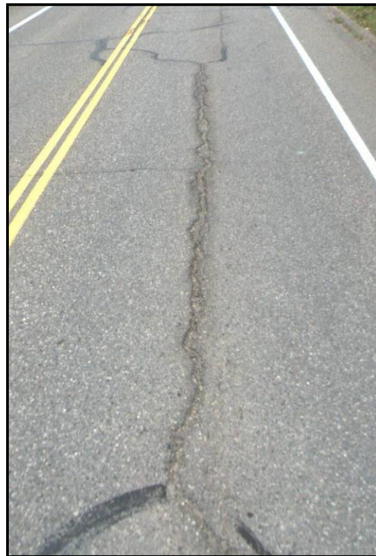
Figure 20 - High Severity MLC
