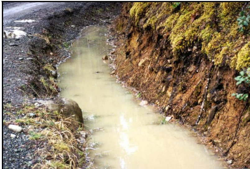
Figure 42 – Unacceptable Drainage
