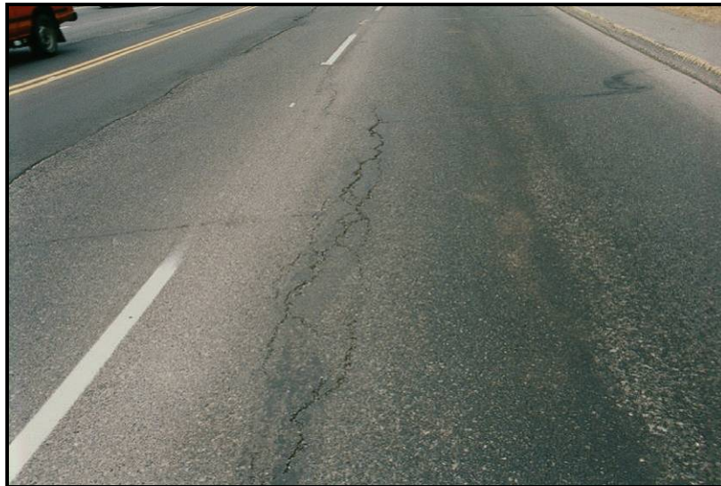
Figure 3 - High Severity LWP (multiple cracks)
