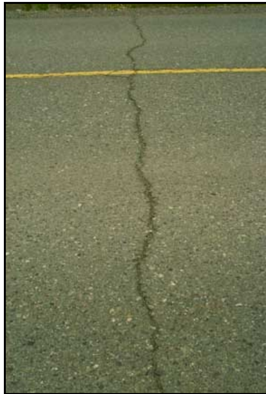
Figure 14 - Moderate Severity TC
