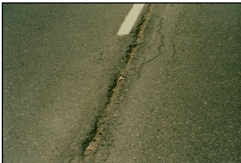
Figure 8 - High Severity LJC (single crack)
