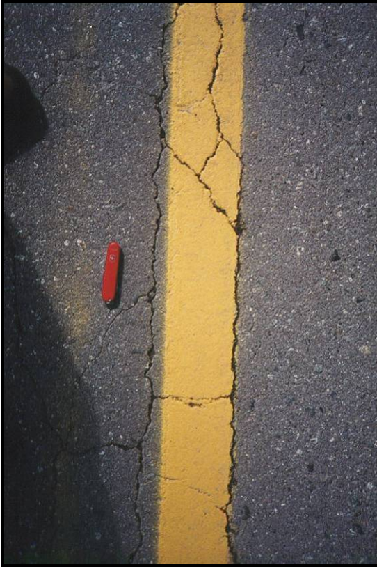
Figure 5 - Low Severity LJC
