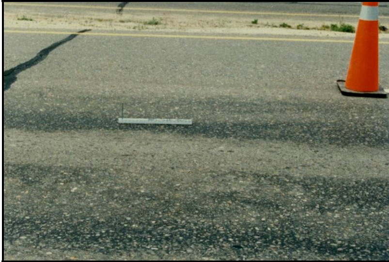
Figure 33 - Moderate Severity BLD
