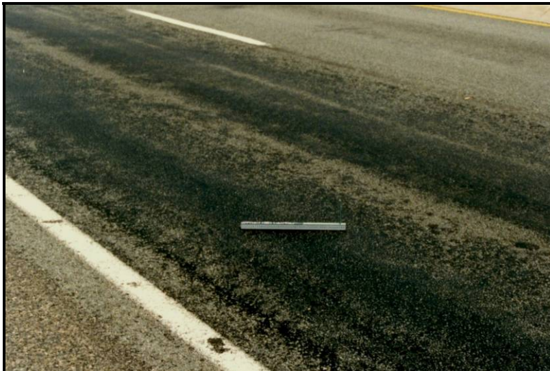
Figure 34 - High Severity BLD
