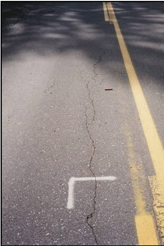
Figure 1 - Low Severity LWP
