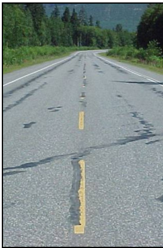
Figure 44 - Level 3 Sealing
