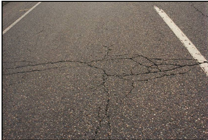
Figure 21 - Moderate Severity AC (progressed from multiple cracks)
