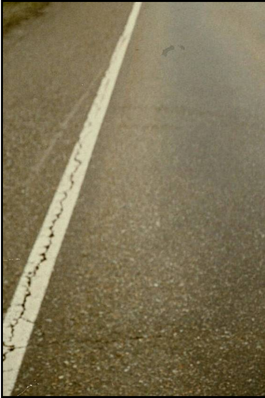
Figure 9 - Low Severity PEC
