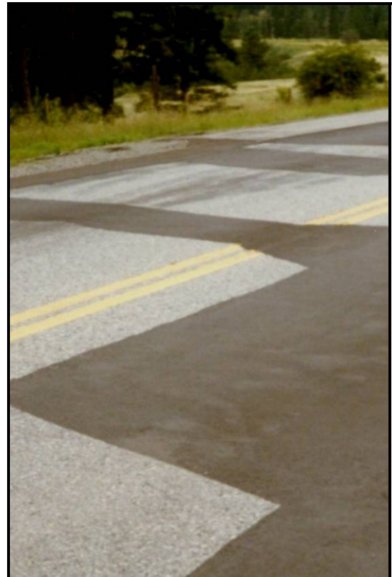
Figure 46 - Level 2 Patching
