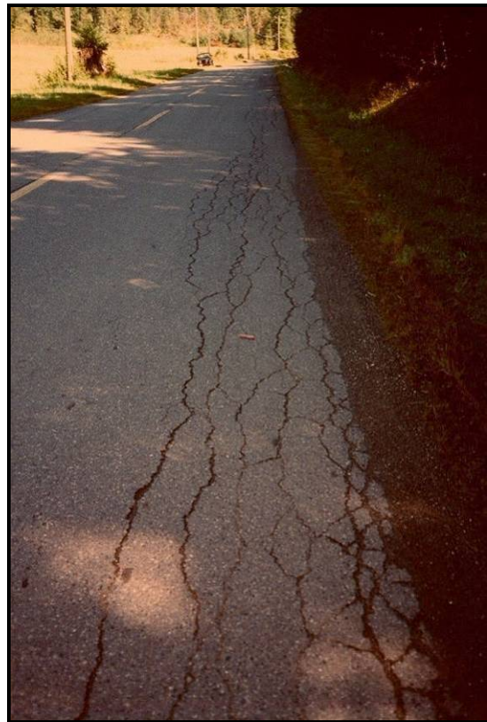
Figure 12 - High Severity PEC
