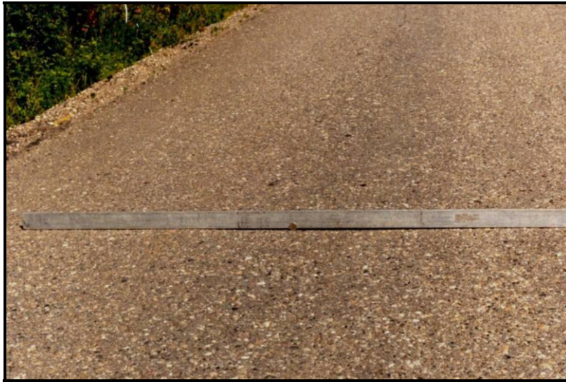
Figure 25 - Low Severity RUT
