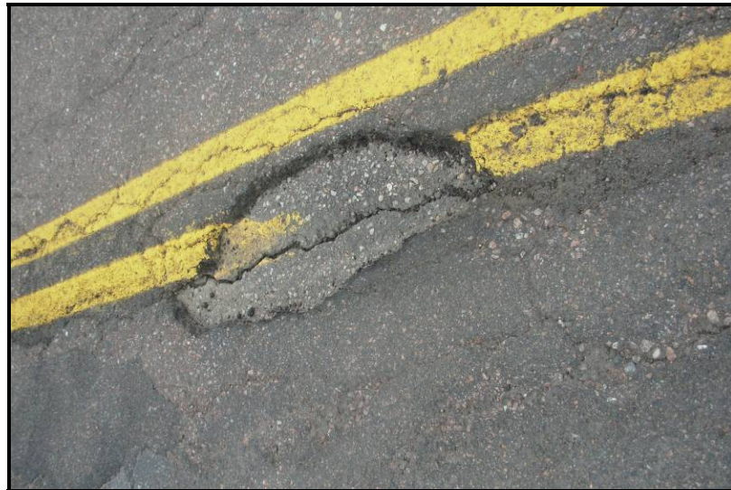
Figure 36 - Moderate Severity POT
