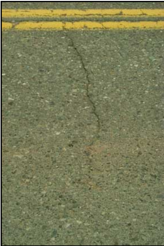
Figure 13 - Low Severity TC
