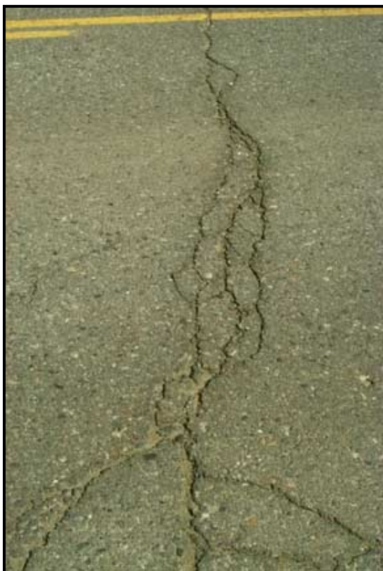
Figure 15 - High Severity TC (multiple cracking and spalling)
