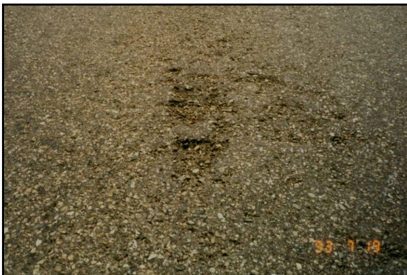
Figure 40 - High Severity RAV
