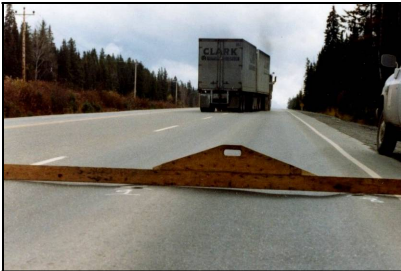
Figure 28 - High Severity RUT
