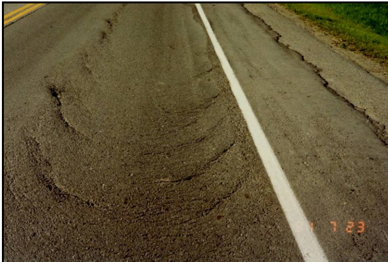
Figure 30 - High Severity SHV (defined by relative effect on ride quality)
