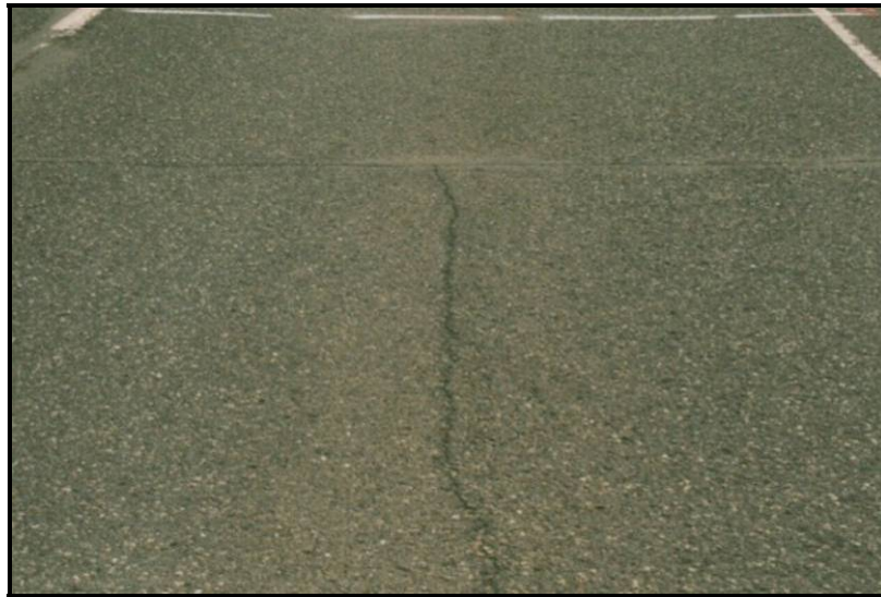
Figure 17- Low Severity MLC
