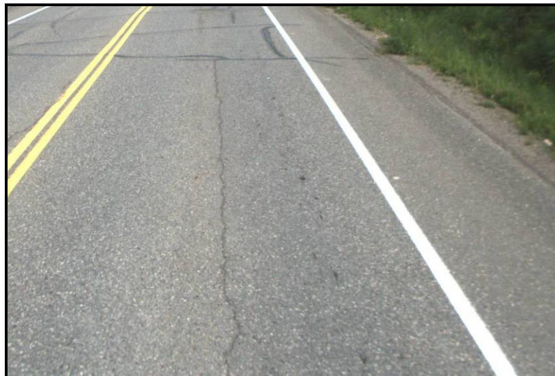
Figure 18 - Moderate Severity MLC
