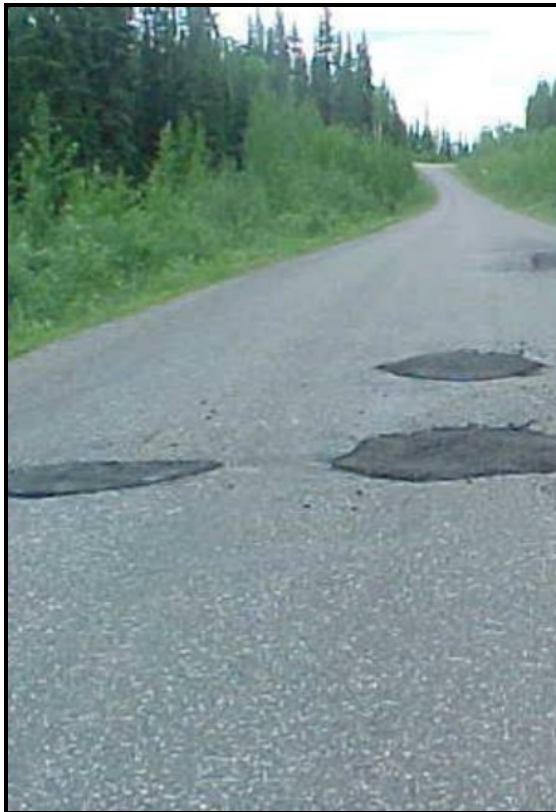
Figure 45 - Level 1 Patching
