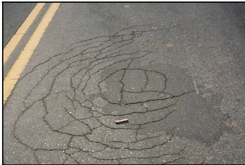
Figure 22 - Moderate Severity AC (localized failure)
