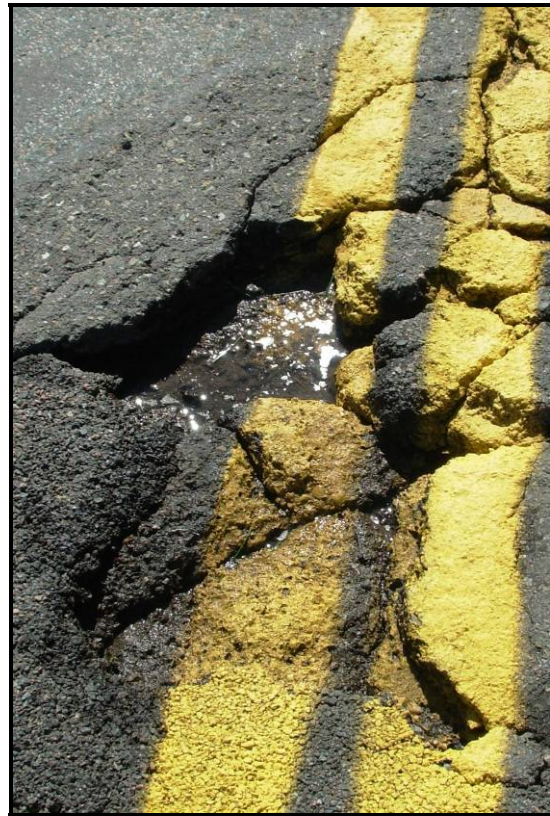
Figure 38 - High Severity Pothole with asphalt break up
