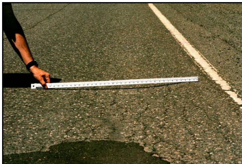
Figure 26 - Moderate Severity RUT
