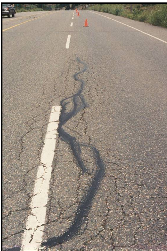
Figure 43 - Level 1 Sealing
