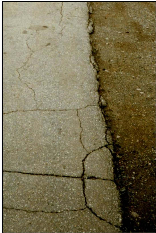
Figure 10 - Moderate Severity PEC
