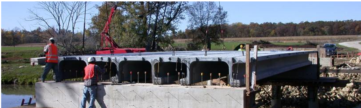
Installation des poutres – pont Buchanan County, Iowa
