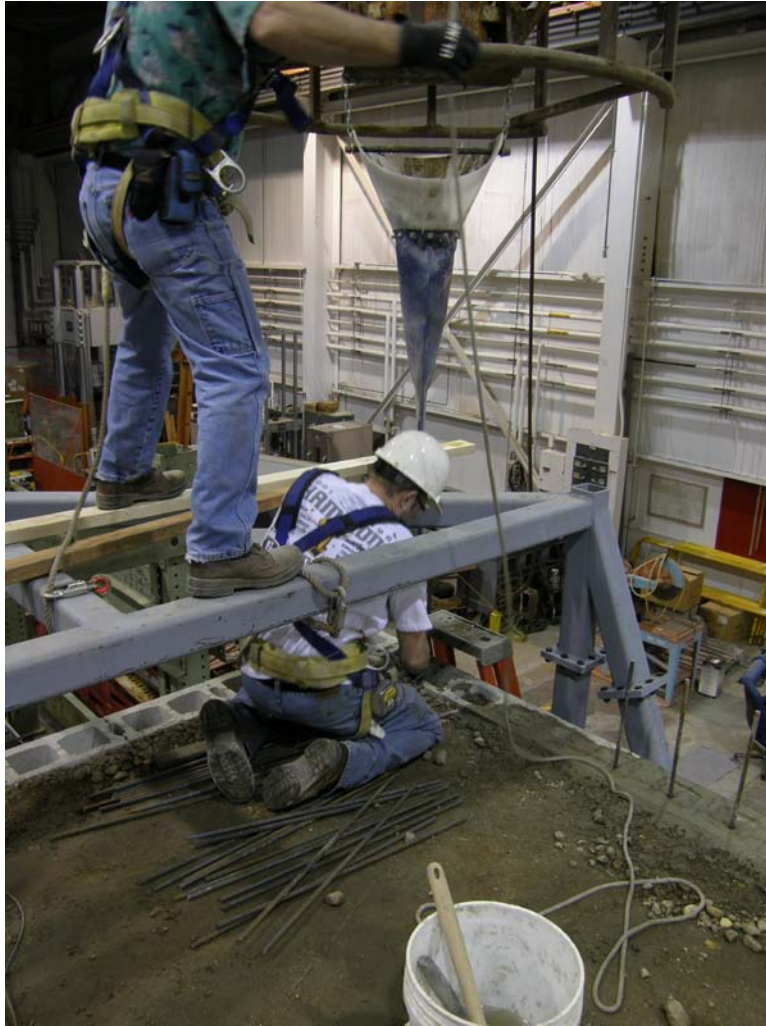
Figure 5.6: Grouting the Top Three Courses of Blocks
