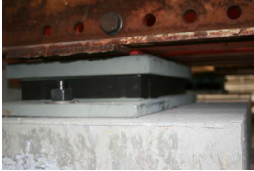
Figure 5.8: Elastomeric Pad Close-up
