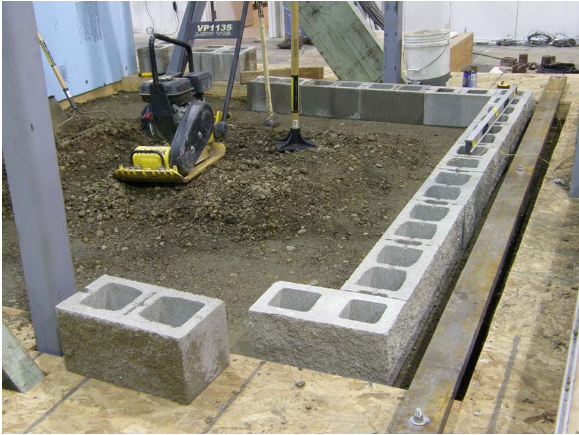
Figure 5.5: First Course of Block Placement
