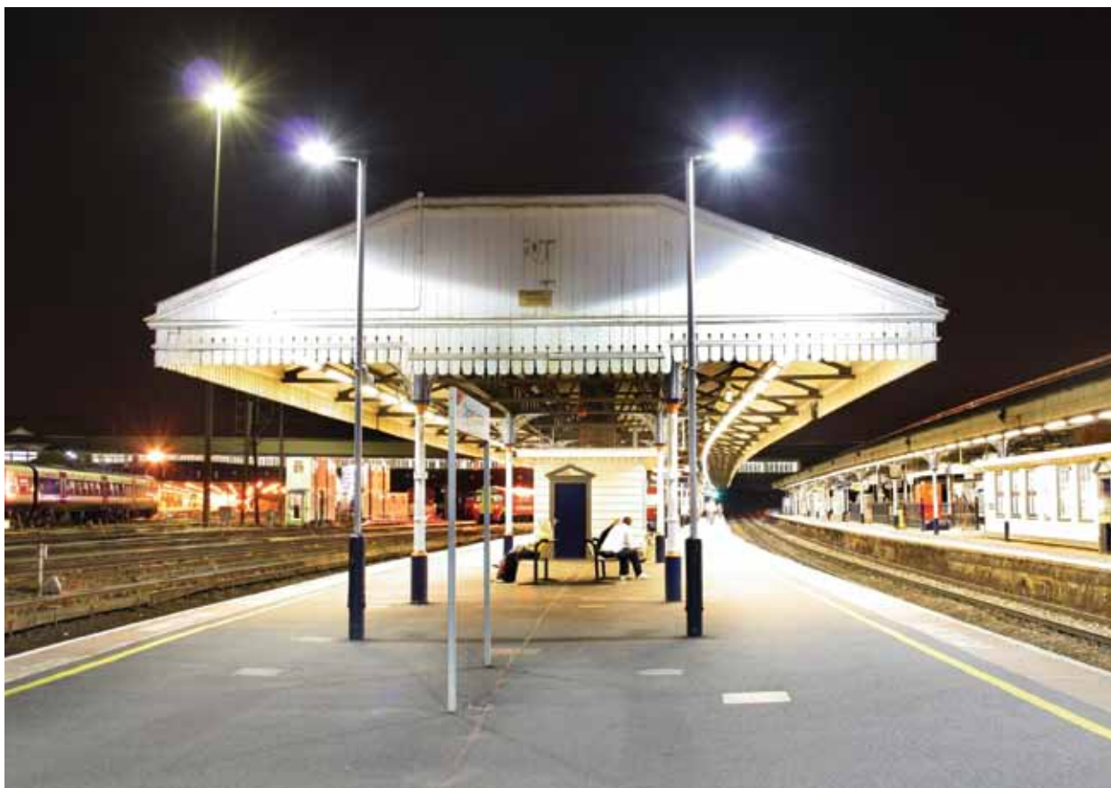
Figure H1.1 Well-lit platforms
