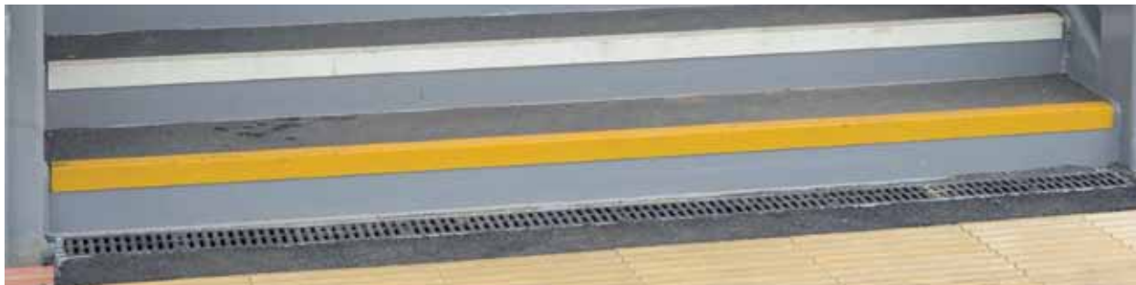
Figure T3.1 Corduroy tactile paving at the bottom of a staircase
