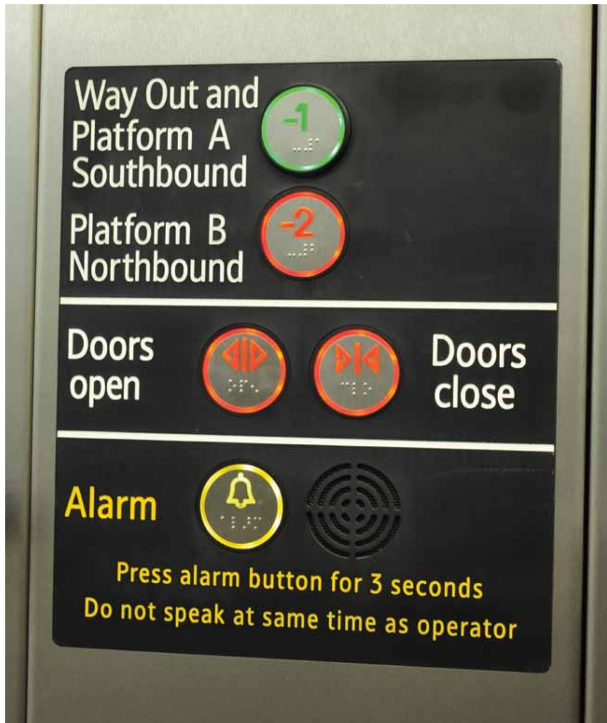
Figure K6.1 Lift control buttons with Braille markings
