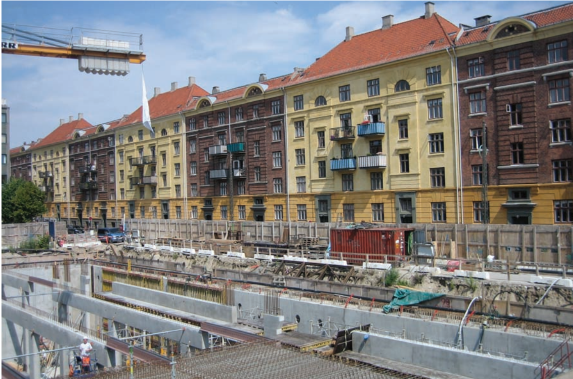
Construction of a 400-space underground parking facility with residential units above, in the Islands Brygge neighborhood of Copenhagen, Denmark.
