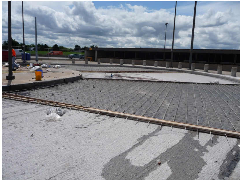
Fig. 9. FRP mat each way – East Transitway, Ottawa, ON 2009
