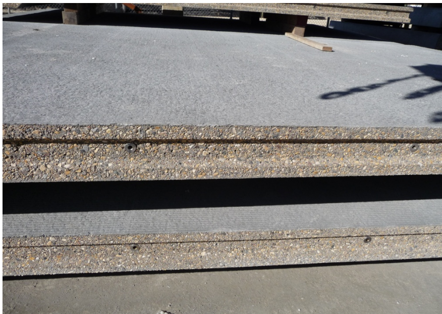
Fig. 10. Top & bottom bar in precast, CFRP prestressed– Noden Causeway ON 2008
