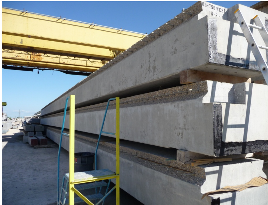
Fig. 12. FRP precast structure Hawk Lake bridge, MTO NW, ON 2008
