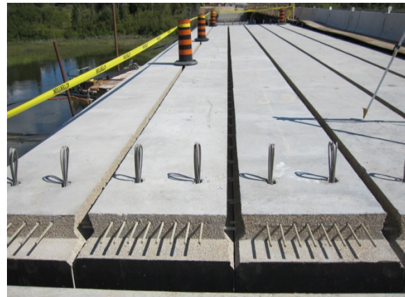
Fig. 4. Finished precast girders – MTO NW region
