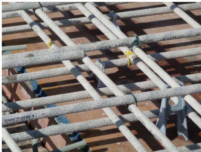
Fig. 1. FRP deck bar ready to cast – Waterloo Region
