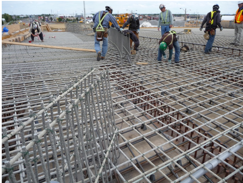
Fig. 6. FRP decks and barriers – Gateway Blvd/23 rd Ave – Alberta 2009
