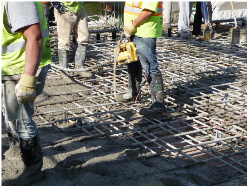
Fig. 8. FRP top & bottom layers of decks – Bridgeport Bridge – Waterloo, ON 2009
