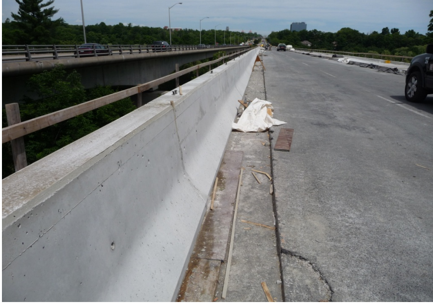
Fig. 11. FRP in barriers – Burnhamthorpe bridges, Mississauga, ON 2009
