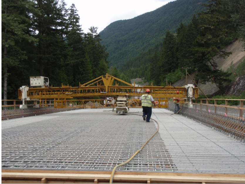
Fig. 7. FRP decks/app slabs/ barriers – Skagit River – BC MOT 2009
