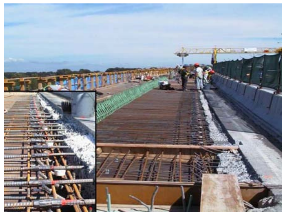
Figure 3: Discrete Anodes Used for Bridge Widening at the Interface Between Old and New Concrete
