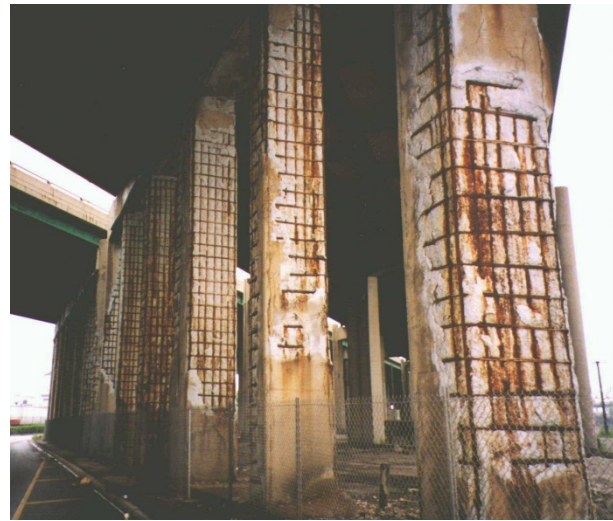
Figure 1: Bridge Columns Damaged by Corrosion of Reinforcing Steel Due to De-icing Chemical Exposure
