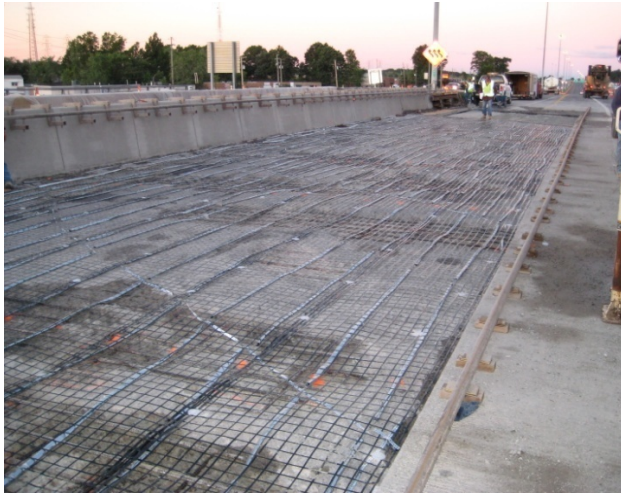
Figure 9: Distributed Anodes Installed on Ohio ODT Bridge Deck
