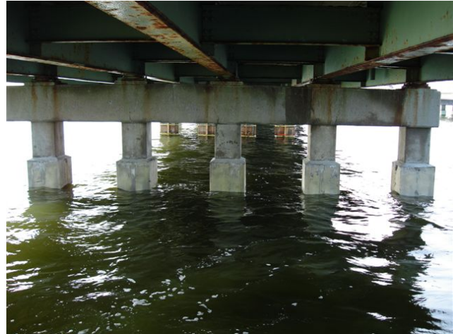
Figure 12: Completed Pile Repair (Galvanic Encasement with FRP Jacket) for New York State DOT
