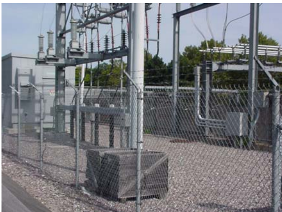
Figure 2-3 - Typical 2x25 kV System Autotransformer Station
