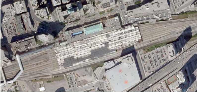
Figure 2-2 – Aerial View of Union Station
