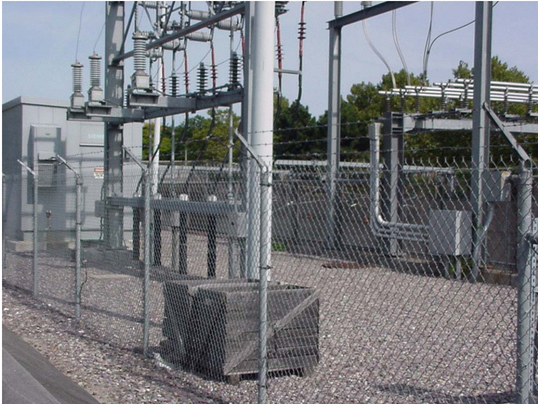
Figure 10: Typical 2x25 kV System Autotransformer Station
