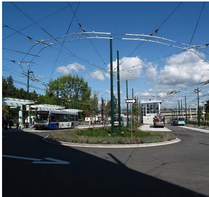
FIGURE 88: TERMINUS À VANCOUVER
