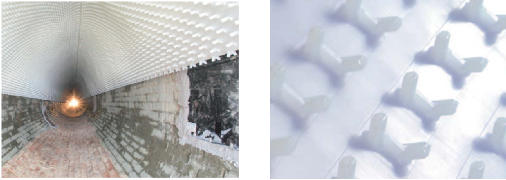
Figure 1. Troliner installed in an egg-shaped brick work sewer sized 1.4 x 2.1 m inner diameter (left); close-up picture of Troliner surface (right).
