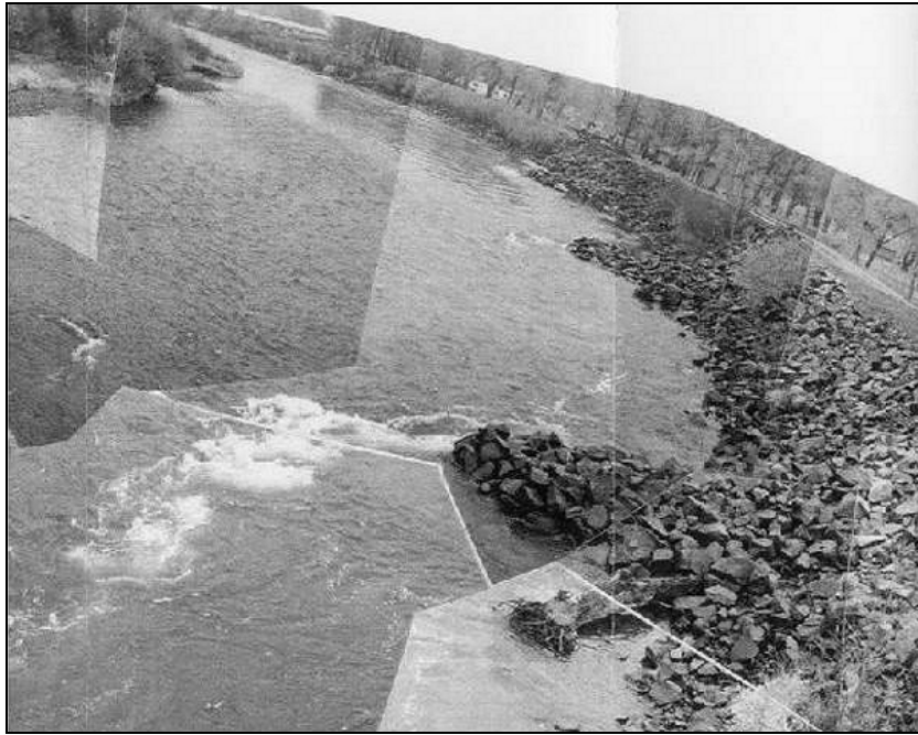
Figure 1.6. Bendway weirs on the Yakima River, Washington at low flow (WSDOT).
