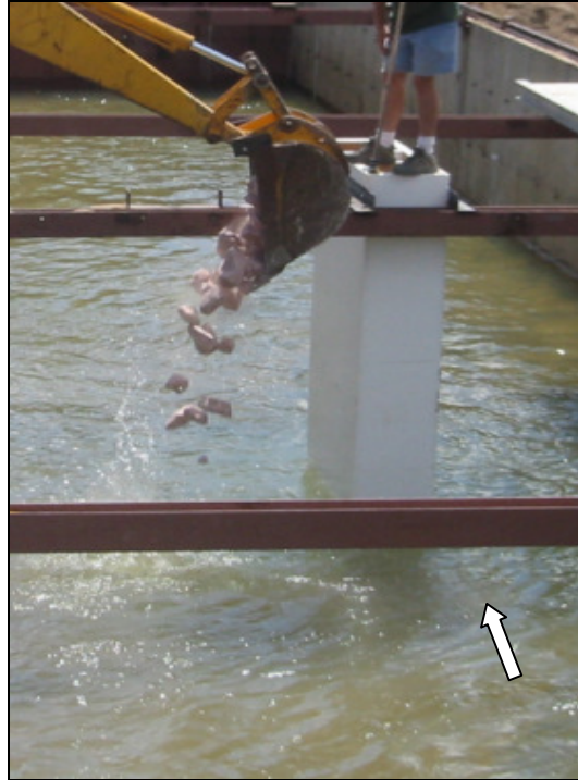
Figure 11.13. Installation of riprap around pier.
