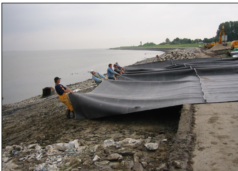
Figure 4.10. Hand placing geotextile prior to placing riprap. Note sewn seam.
