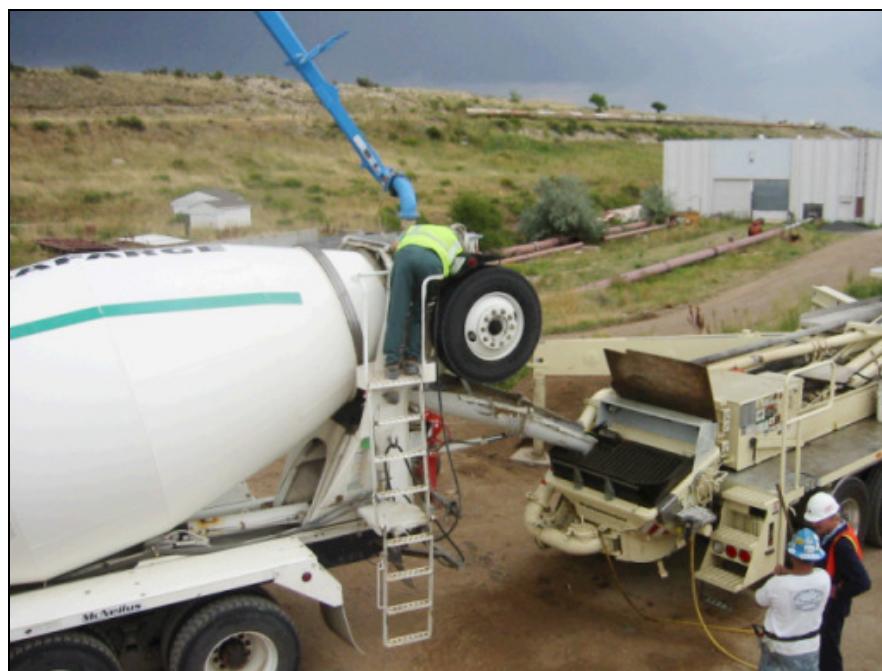
Figure 12.7. Concrete mixer truck and pump truck with boom.
