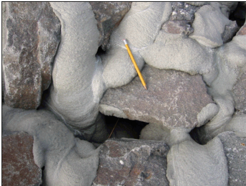
Figure 12.1. Close-up view of partially grouted riprap.
