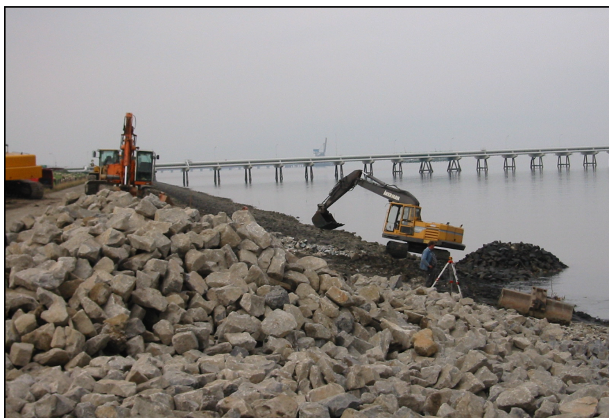
Figure 4.11. Placing riprap with hydraulic excavators.
