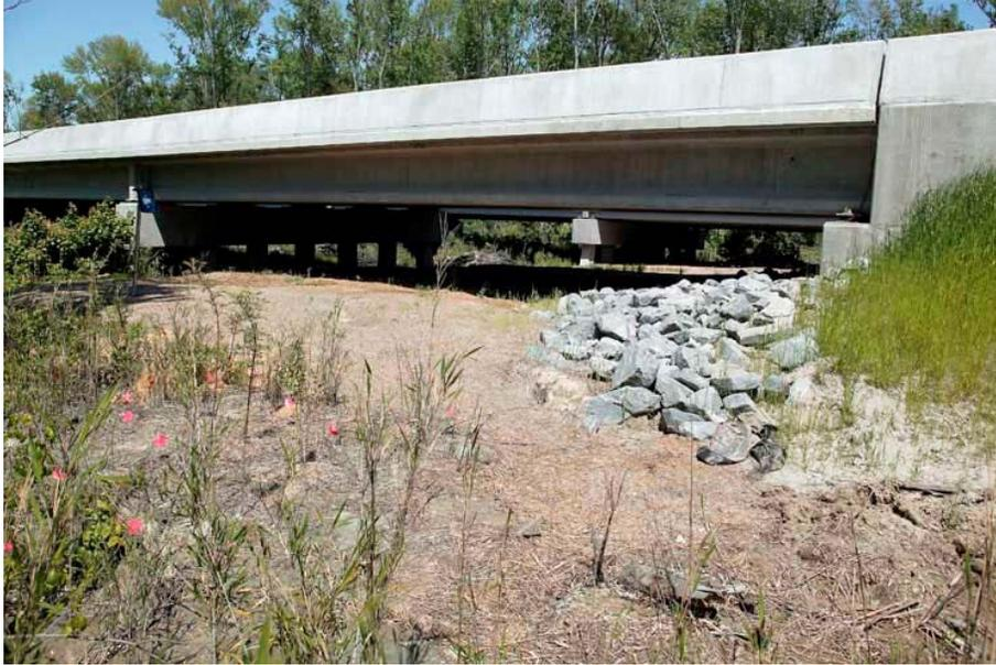
**Figure 2. U.S. Highway 17 Underpass. The underpass is 984 ft wide (from the animal’s perspective) and spans 4 lanes and an open median. The photograph illustrates one of the dry areas (berms) that was constructed at each end of the underpass, intended for use by wildlife.**
