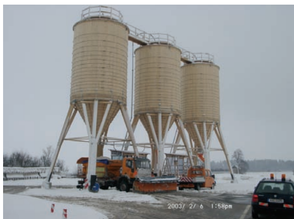
Optimizing time for loading by using salt storage silos
