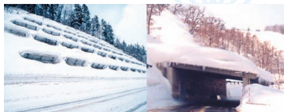
Avalanche control fence
