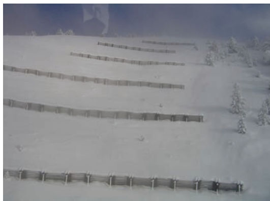
10- Protective barriers, screens, Nicolau Canal, El Serrat.
