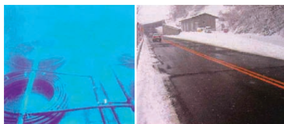
Underwater spiral coils Snow melting with the system
