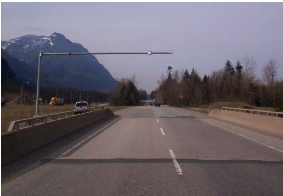
Figure 6: Photograph of Green Light Transportation System site at Hunter Creek
