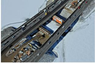
Figure 29 – WB Bridge False Deck
