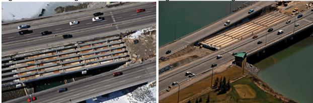
Figure 31 – WB Bridge Deck Pour
