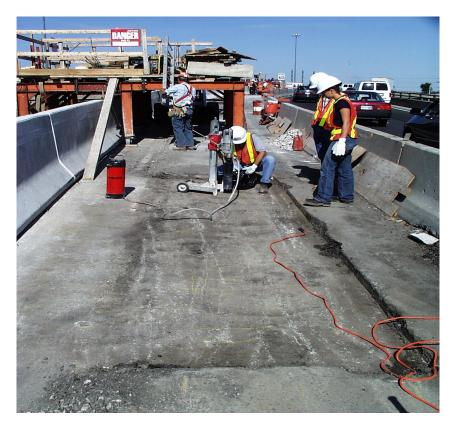
Figure 9 Condition Survey on Latex Modified Concrete Overlay 2002 (QEW/Hwy 427 Bridge No. 7)
