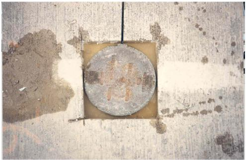
Figure 3 Pancake anode recessed into concrete deck
