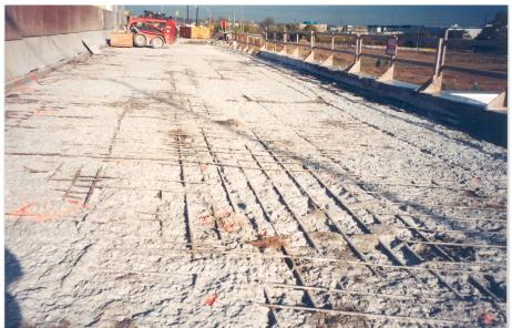
Figure 14 Top surface of deck after hydrodemolition, Hwy 25 over Hwy 401
