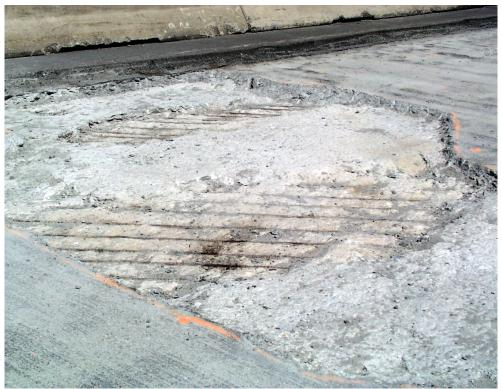
Figure 11 Localized corrosion of rebars over circular voids of PT deck
