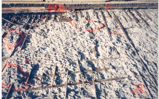
Figure 15 Condition of reinforcing steel after hydrodemolition
