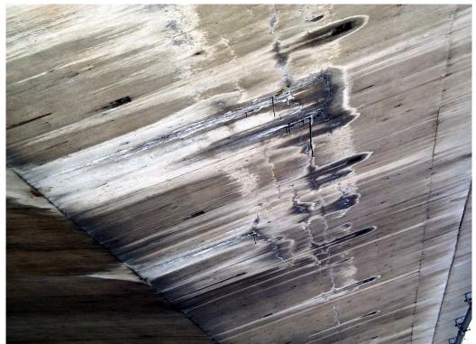
Figure 6 Soffit of Post-Tensioned Deck with leaching cracks
