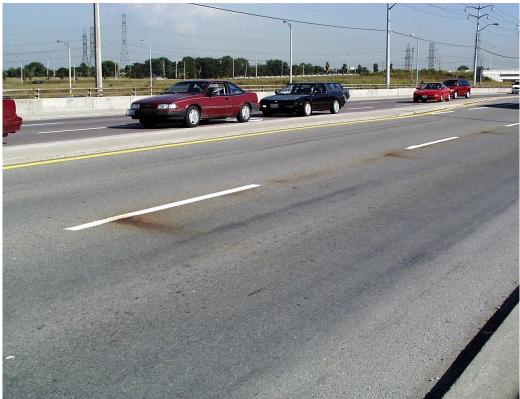
Figure 7 Rust staining at anodes of conductive asphalt CP system
