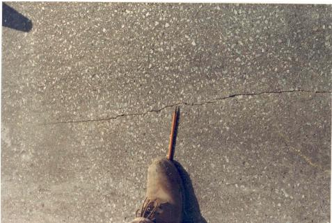
Figure 1 QEW WB to Highway 427 SB Ramp (Photo taken 1989) - Typical longitudinal crack in deck over voids
