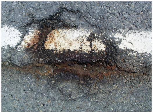
Figure 8 Asphalt deterioration at anode of conductive asphalt CP System
