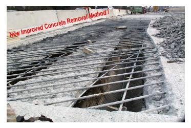
Figure 16 Excessive concrete removal of a post-tensioned deck with circular voids
