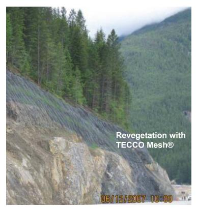
**Figure 3.** Example of TECCO Mesh® used to stabilize and assist revegetation of steep slopes on Phase 2 of the Kicking Horse Canyon Project.
