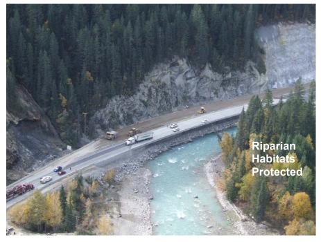
Figure 5. Cantilevered structure along the Kicking Horse River reduced further riparian impacts.
