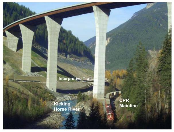
Figure 6. Park Bridge is a full span structure that avoids instream impacts to the river.
