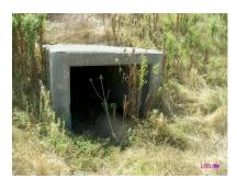
Figure 0.2 Concrete Box Culvert, Kitchener
