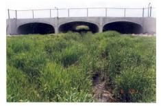
Figure 0.4 Multi-Cell Pre-cast Open Bottom Culvert, Markham
