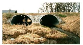
Figure 0.3 Open Arch-style Culvert – Double Cell
