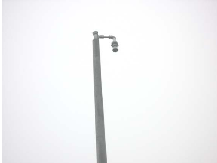
Figure 6 – Dome CCTV Camera on EC Row
