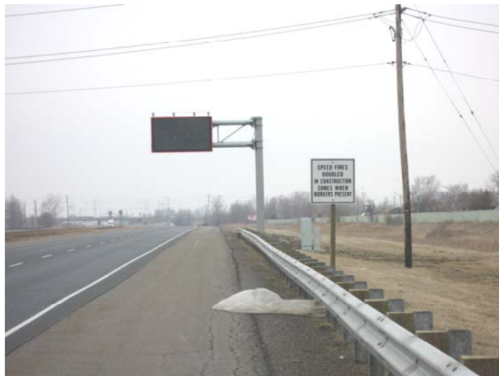
Figure 7 - Cantilever Variable Message Sign on EC Row
