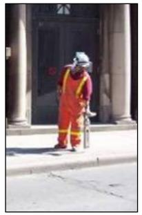
Figure 3 - Field Technician using Cable Locate Equipment
