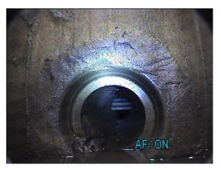
Figure 6 - Zoom Camera photo showing conduits directionally drilled through Storm Sewer
