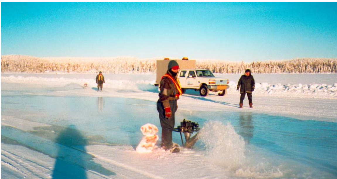
FIGURE 8 Ice Flooding Activities to Increase Ice Sheet Thickness.
