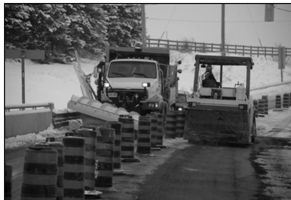
Figure 8d: Intermediate Rolling of Mix
