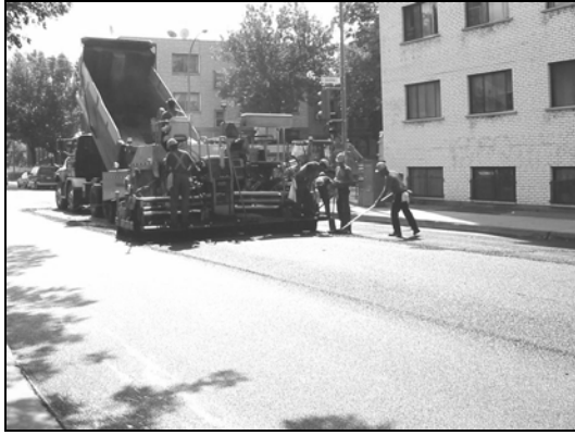
Figure 1: Warm Mix Placement on Rue Ball in August 2005 and One Year Later
