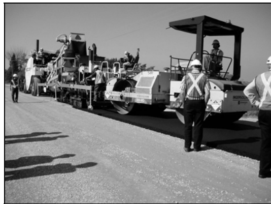
Figure 4b: Warm Mix Placement
