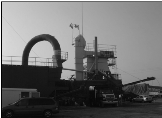
Figure 4a: Ramara Plant
