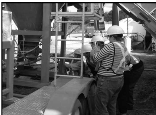
Figure 2: Zeolite Injection and Laydown of Aspha-min® Warm Mix on Autoroute 55
