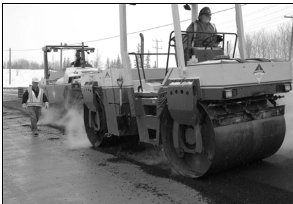
Figure 8c: Breakdown Rolling of Mix
