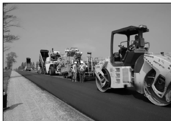
Figure 7d: Laydown of DAT
