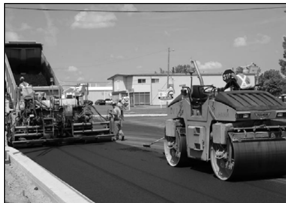
Figure 5b: Warm Mix Placement
