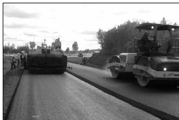
Figure 2: Zeolite Injection and Laydown of Aspha-min® Warm Mix on Autoroute 55
