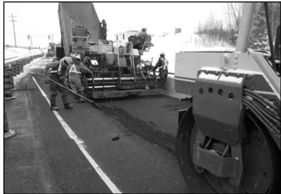
Figure 8b: Placement on Bridge deck
