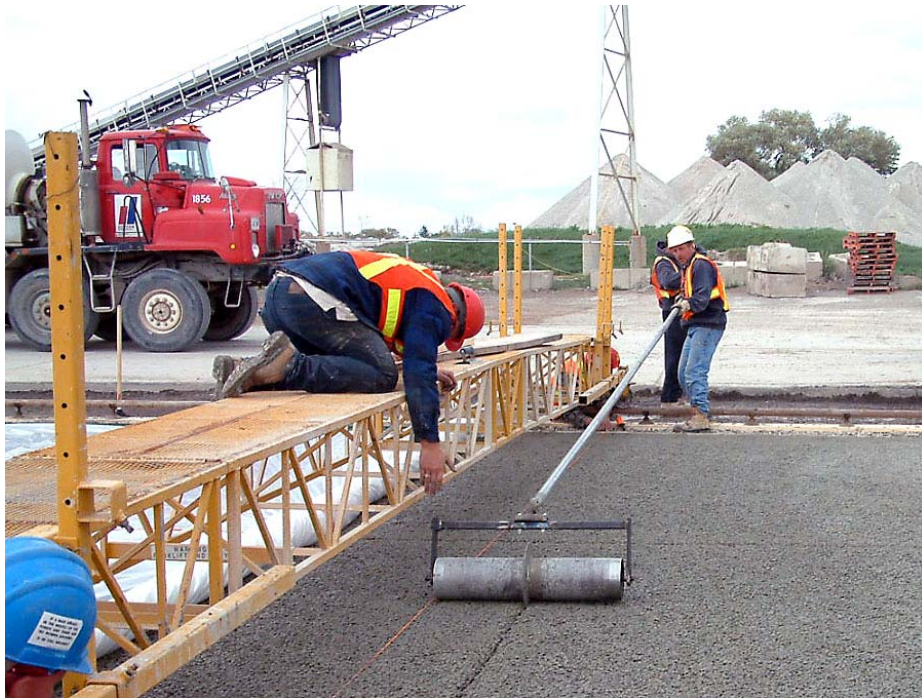
Figure 3. Transverse Joint Rolling (Trial Slab)
