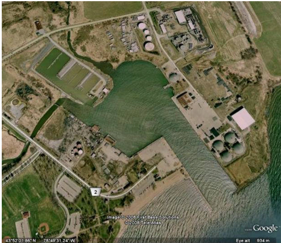
Figure 1. Aerial View of the Port of Oshawa
