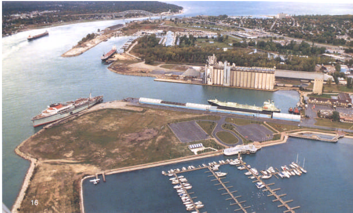
Figure 11. Transport Canada’s Facilities at Sarnia
