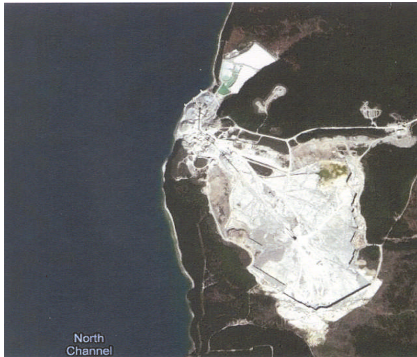
Figure 14. Harbour of Meldrum Bay
