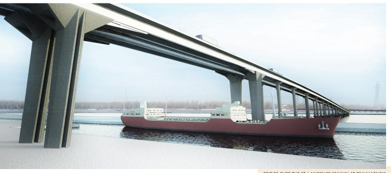
The bridge that crosses the St. Lawrence River over a distance of almost two kilometres between Les Cèdres to the north and Salaberry-de-Valleyfield to the south will be designed with a harmonious set of piles that will rise progressively under a standard highway structure.
