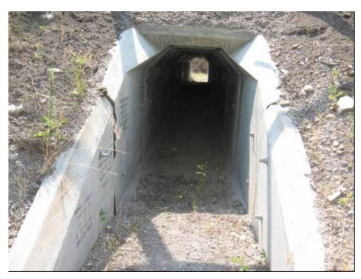
Figure 48. A medium-mammal box culvert (1.2 m (3.9 ft) wide, 1.8 m (5.9 ft) high) along U.S. Highway 93, south of Ravalli, MT (copyright: Marcel Huijser).
