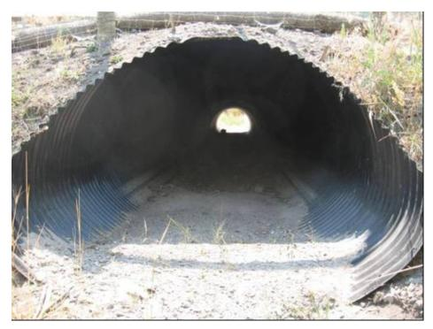
Figure 49. A medium-mammal culvert (2 m (6.6 ft) wide, 1.5 m (4.9 ft) high) along U.S. Highway 93, south of Ravalli, MT (copyright: Marcel Huijser).
