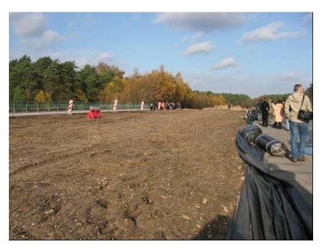
Figure 89. Road removed on bridge over motorway in Belgium and replaced with soil for vegetation and bike path (copyright: Bethanie Walder).
