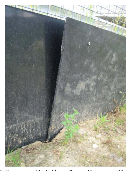
Figure 116. Plastic screens combined with a medium- and large-mammal fence guiding the animals toward an overpass (Waterloo) along the A73 motorway near the town Roermond, The Netherlands. Note that the screw that holds the two plastic sheets together is broken, allowing for a gap and potential intrusions of amphibians and other small species into the road corridor (copyright: Marcel Huijser).
