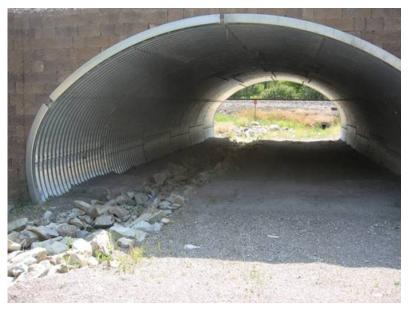
Figure 73. Wildlife underpass (large-mammal culvert) along U.S. Highway 93 in Montana with a ditch that allows water to flow (seasonally) (copyright: Marcel Huijser).
