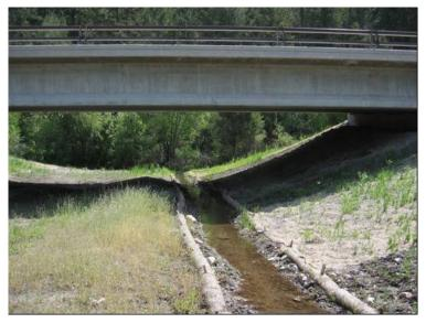
Figure 74. Wildlife underpass (over-span bridge) in combination with a creek crossing along U.S. Highway 93 in Montana (copyright: Marcel Huijser).
