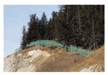
Figure 36. A 2.4-meter-high (8-ft-high) large-mammal chain-link fence along the Trans-Canada Highway between Canmore and Banff, Alberta, is equipped with green mesh to make the fence more visible to bighorn sheep (copyright: Marcel Huijser).
