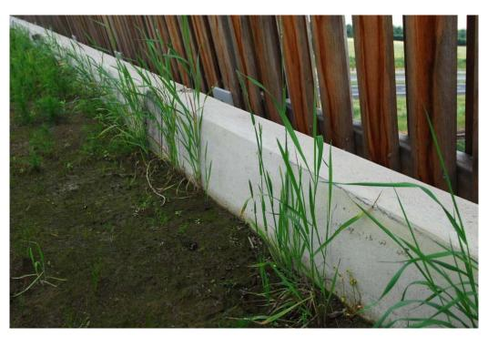
Figure 64. The wildlife fencing on the wildlife overpass "Waterloo" across the A73 motorway near the town "Roermond", The Netherlands. Note that the concrete barrier prevents small animal species from falling off the overpass (copyright: Marcel Huijser).
