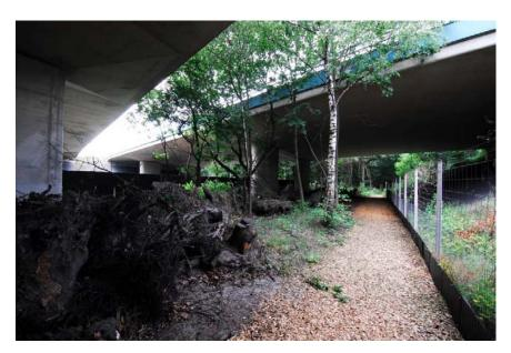
Figure 82. An underpass for a road (Hilversumsestraatweg) under the motorway A27 near the town "Hilversum", The Netherlands, that was modified with soil and tree stumps to encourage co-use by wildlife. Note that light and moisture allow for shrubs and trees in the gap in the median (background) and that tree stumps provide cover under the bridge for northbound traffic (foreground) (copyright: Marcel Huijser).
