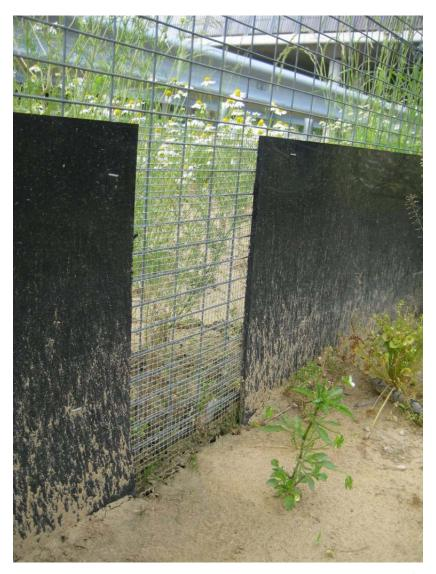
Figure 117. Plastic screens combined with a medium- and large-mammal fence guiding the animals toward an overpass (Waterloo) along the A73 motorway near the town Roermond, The Netherlands. Note that two adjacent sheets have a gap that is covered by fine mesh wire fence to prevent amphibians and other small species from entering the road corridor (copyright: Marcel Huijser).
