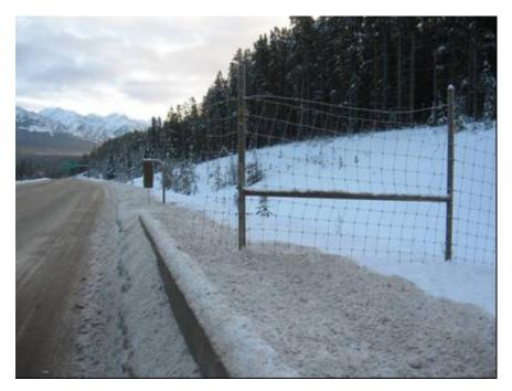
Figure 27. Fence end brought close to the road with a concrete barrier for safety in Banff National Park, just west of Castle Junction, Alberta (copyright: Marcel Huijser).
