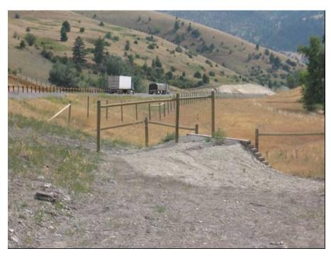
Figure 30. A short section of perpendicular fence to guide animals on top of a jump-out along a 2.4-meter-high (8-ft-high) fence along U.S. Highway 93 in Montana (copyright: Marcel Huijser).
