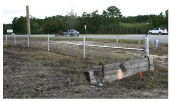
Figure 110. Fences keep Alabama red-bellied turtles from entering the roadway and lead them toward bridges where they can cross under the road (copyright: ALDOT).
