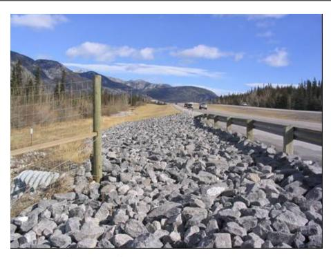
Figure 28. The boulder field at the fence end at Dead Man's Flats along the Trans-Canada Highway east of Canmore, Alberta (copyright: Bruce Leeson).
