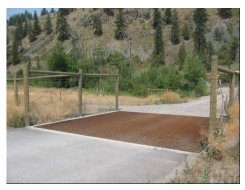
Figure 39. A modified wildlife guard (bridge-grate material) at an access road on U.S. Highway 93, south of Ravalli, MT (copyright: Marcel Huijser).
