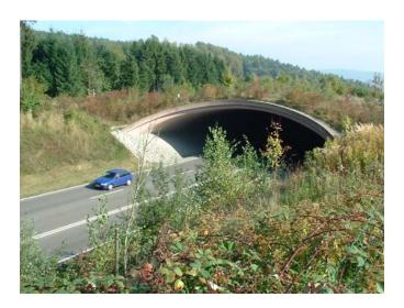
Figure 60. A wildlife overpass in Germany. The terrestrial habitat connected by the overpass is at a higher elevation than the roadway (copyright: Mary Gray, FHWA).
