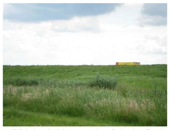
Figure 137. Embankment for birds to encourage them to fly above the traffic on the A27 motorway near Huizen, The Netherlands. Embankments are on both sides of the road, and also serve to reduce sound and light disturbance into the open grasslands. Note that the yellow top of a freight truck shows just above the embankment (copyright: Marcel Huijser).
