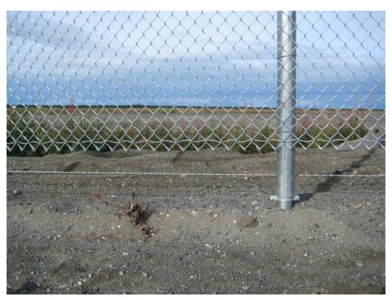
Figure 24. A chain-link moose fence near Kenai, AK, with a gap (and a barbed wire strand) at the bottom allowing small species to crawl underneath the fence (copyright: Marcel Huijser).
