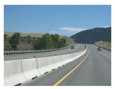
Figure 8. Long sections of median barriers are thought to increase road mortality and reduce animal movements across the road. Note that the small cutouts at the bottom of concrete median barrier are designed for drainage but also allow small animal species to cross under the median barriers (copyright: Marcel Huijser).
