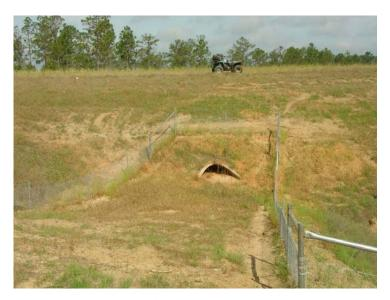
Figure 109. Fences lead gopher tortoises toward a culvert along Highway 63 in Green County, south of Leakesville, MS (copyright: Chuck Walters).
