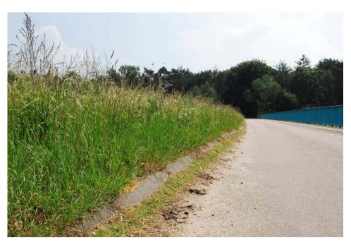
Figure 86. The same overpass as figure 85 showing the gentle grade of the concrete curb, which allows small animals to access the vegetated strip (copyright: Marcel Huijser).
