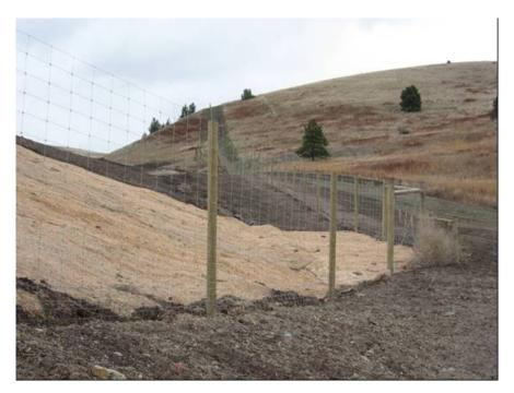
Figure 57. After construction, straw mats were used to protect slopes from erosion and rapid establishment of weeds along U.S. Highway 93 in Montana (copyright: Marcel Huijser).
