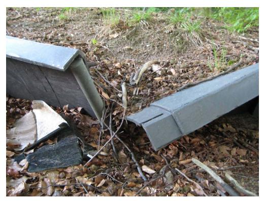
Figure 118. Plastic screens that collapsed were intended to guide amphibians toward an underpass near the town Hilversum, The Netherlands. The gap allows amphibians and other small species to enter the road corridor (copyright: Marcel Huijser).
