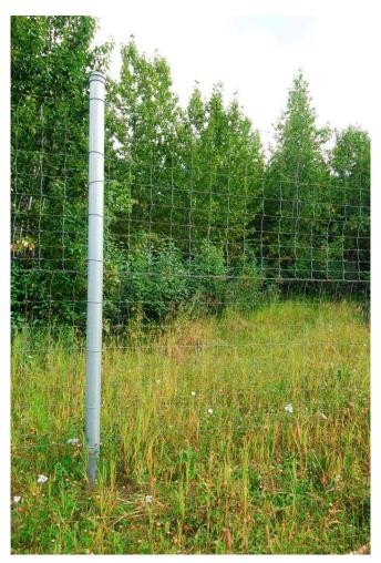
Figure 15. A moose fence, along the Glenn Highway (Hwy 1), northeast of Anchorage, AK (copyright: Marcel Huijser).
