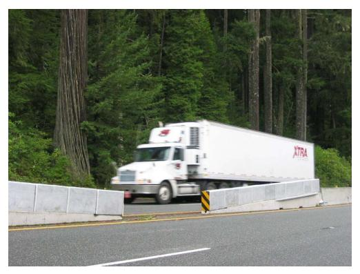
Figure 10. Opening in median barriers designed to allow wildlife to cross the road and the median barriers (copyright: Marcel Huijser).
