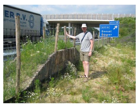
Figure 32. A jump-out intended for Eurasian badger and roe deer along a 2-meter-high (6.6-ft-high) fence along the A73 motorway near Roermond, The Netherlands. Note the wildlife overpass "Waterloo" in the background (copyright: Marcel Huijser).
