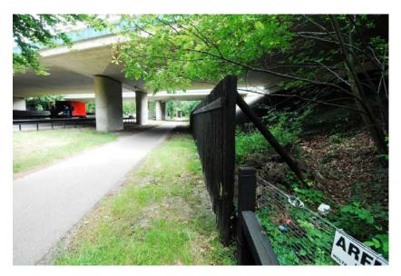
Figure 83. An underpass for a road (Hilversumsestraatweg) under the motorway A27 near the town "Hilversum", The Netherlands, that was modified with soil and tree stumps to encourage co-use by wildlife to the right of the fence. The purpose of the fence, which is painted black, is to reduce light and noise disturbance from traffic (copyright: Marcel Huijser).
