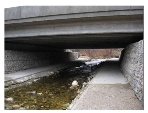
Figure 77. Concrete walkways for wildlife on both banks of a creek at an over-span bridge along U.S. Highway 93, south of Missoula, MT (copyright: Marcel Huijser).
