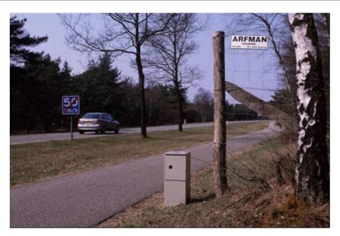
Figure 93. An infrared break-the-beam animal detection system (manufactured by Calonder Energy, Switzerland) at a gap in a wildlife fence near the town 't Harde, The Netherlands (copyright: Marcel Huijser).
