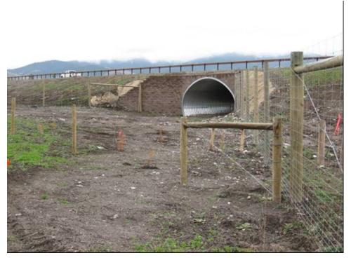
Figure 56. A wildlife underpass with livestock fencing along U.S. Highway 93 in Montana (copyright: Marcel Huijser).
