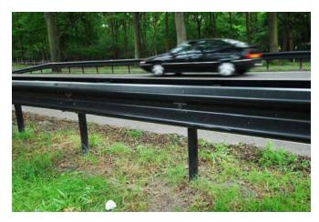
Figure 130. Guardrail painted black near amphibian tunnels and a multiple-use underpass, along the road "Hilversumsestraatweg", near the town Hilversum, The Netherlands. The painted guardrail is expected to reduce glare and light disturbance for amphibians and other species groups (copyright: Marcel Huijser).
