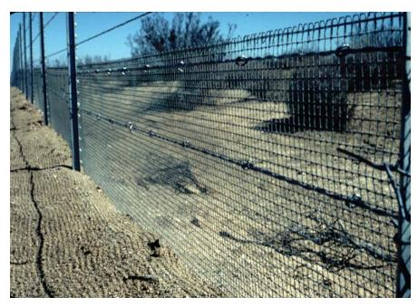
Figure 107. Tortoise barrier fence erected along State Highway 58 near Kramer Junction, San Bernardino County, CA (copyright: William I. Boarman, U. S. Geological Survey).
