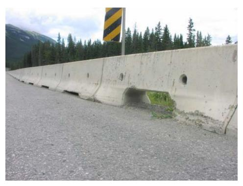
Figure 9. Concrete barriers with scuppers that allow small and mid-sized species to cross under the median barriers (copyright: A.P. Clevenger).
