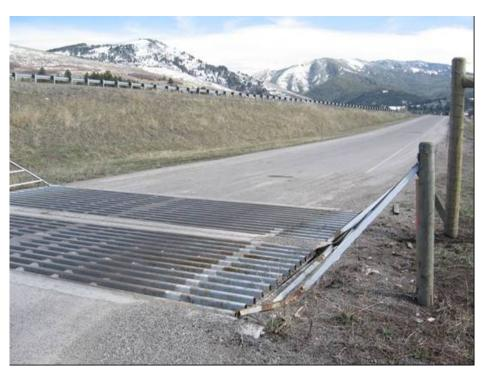
Figure 37. A wildlife guard, similar to a standard cattle guard, at an on-ramp to Interstate 90 east of Bozeman, MT (copyright: Marcel Huijser).
