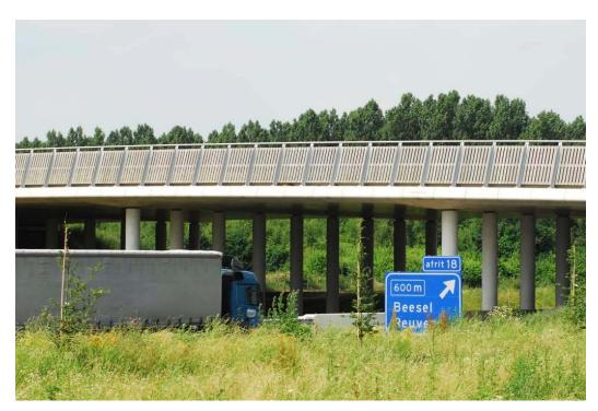
Figure 62. The wildlife overpass "Waterloo" with wildlife fencing across the A73 motorway near the town "Roermond", The Netherlands, consists of planks that also act as a light and sound barrier (copyright: Marcel Huijser).
