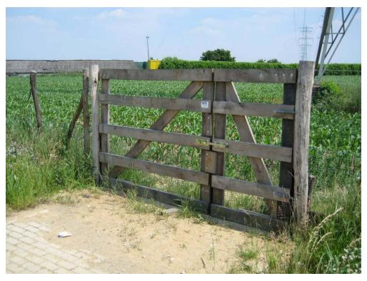
Figure 127. A gate that allows for access to a field with crops through an amphibian barrier, and a medium- and large-mammal fence, near wildlife overpass "Schinheuvel," near the town Roermond, The Netherlands. Note that the gate connects closely to a hard surface to prevent amphibians and other small species from entering the road corridor. (copyright: Marcel Huijser).
