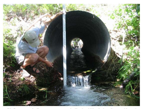
Figure 70. Structures built to pass water typically should be designed to avoid erosion and allow passage of aquatic species. The structure shown has no adaptations for terrestrial species and is also likely to be impassable for many aquatic species (copyright: Matt Blank).
