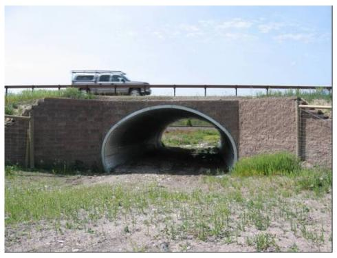
Figure 52. Wildlife fencing ties in with the underpass wing walls, preventing animals from entering the road corridor (copyright: Marcel Huijser).
