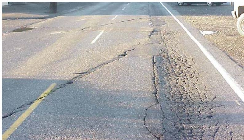
Figure 14. An example of fatigue cracking (Courtesy of the Washington Asphalt Pavement Association)
