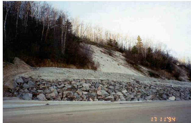
Enrochement et contrepoids, Pointe Lebel, Côte Nord
