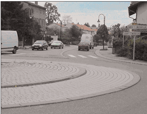
Example of a crown that can be crossed by HGVs inside a roundabout.
