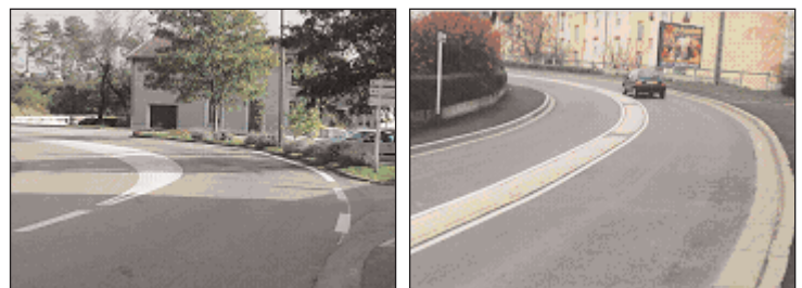
Examples of axial curb lanes that can be crossed by HGVs.
