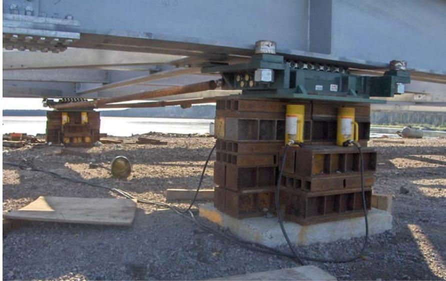
**PHOTO D'AJUSTEMENT D'UN APPUI EN RIVE**
