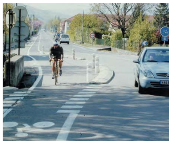
A chicane breaks the straight line of travel but islands ensure the space reserved for cyclists is seamless (FFCT J. Fournia)
