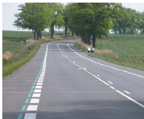
In the Lower Rhine, a green band supplements the white road marking
