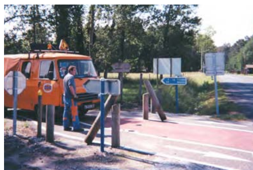
Maintenance operation on a greenway (Cete S.O.)
