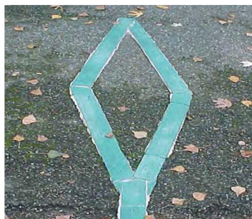
The cycle detector is linked to a magnetic loop (ZELT)
