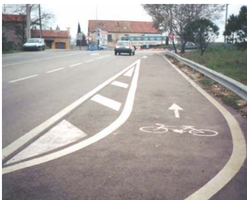
Separation can be made depending on the case, by a refuge island or a hatched area (Certu)
