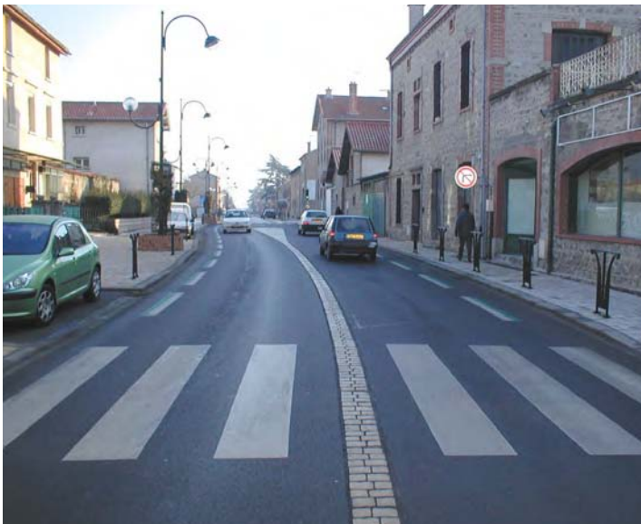
Only if there is little traffic because of limited clearance for overtaking and car doors opening (DDE 42)
