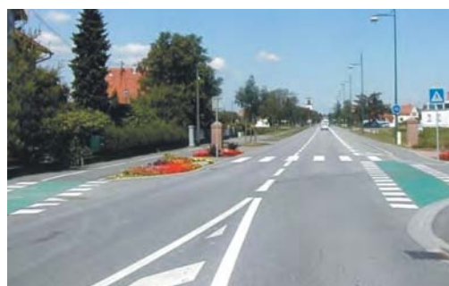
Cycle lane outside a conurbation turns into a cycle path inside the conurbation
