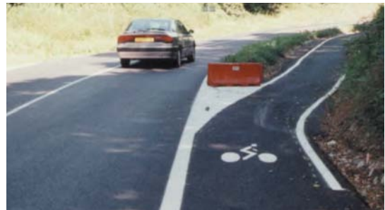
The lane turns into a path on ascending bends (FFCT)
