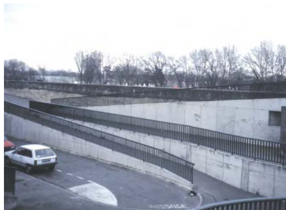
The bridge is accessible to persons with reduced mobility by a ramp with landings (ST Toulouse)
