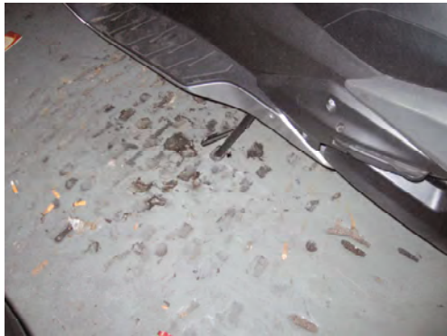
A surface dressing with many damage marks.
