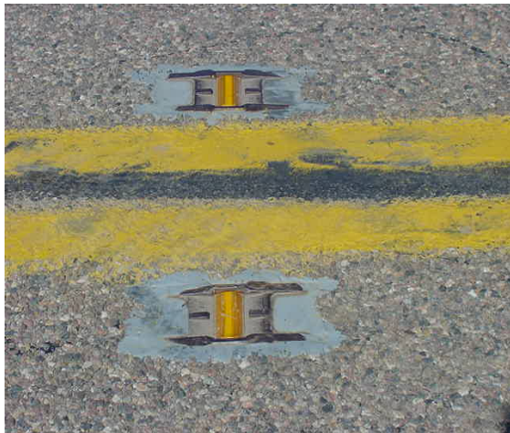
Intact Stimsonite markers at centerline
