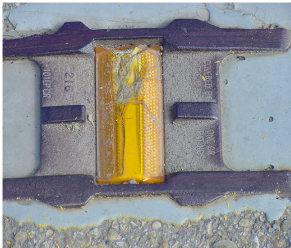
Broken centerline marker
