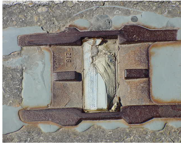
Broken shoulder reflector
