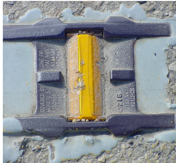
Cracked centerline marker
