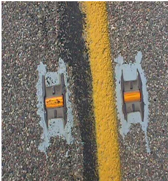
Stimsonite centerline yellow markers Showing crack sealant
