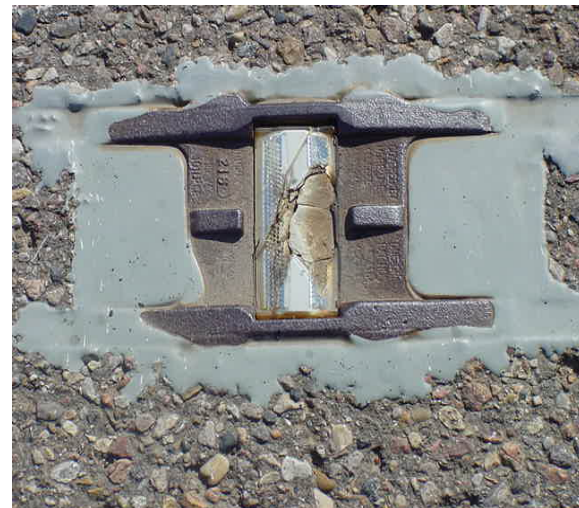
Broken stimsonite marker at shoulder
