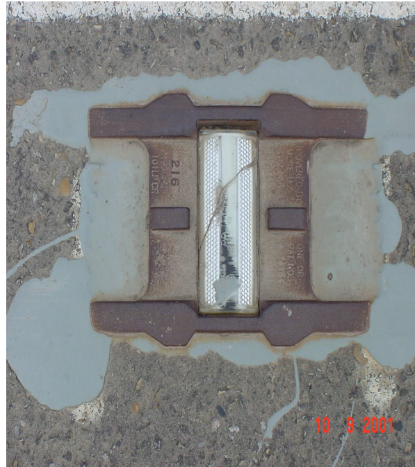
Cracked Stimsonite marker
