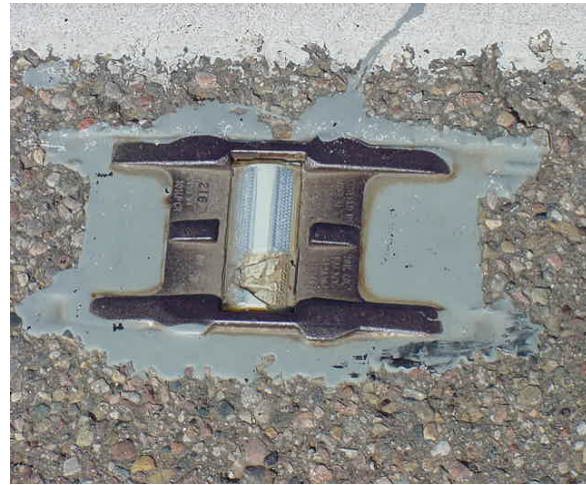
Damaged Stimsonite reflector
