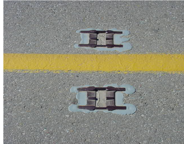
Missing centerline reflectors
