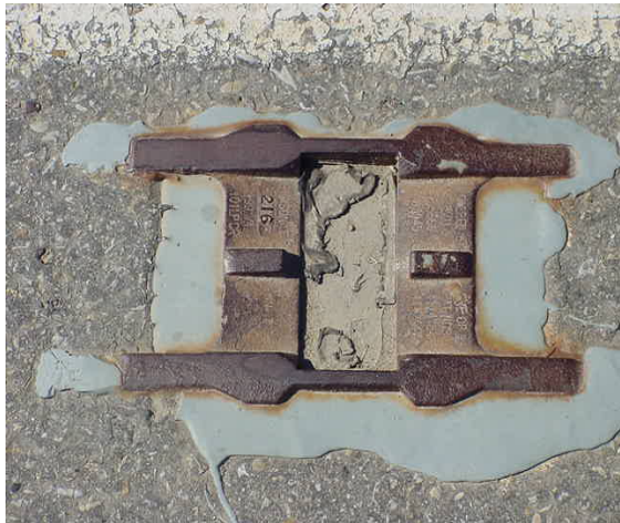
Missing shoulder reflector
