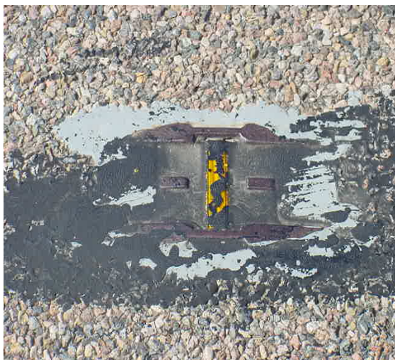
Centerline marker covered with crack sealer
