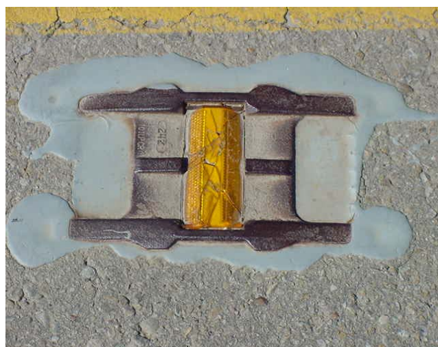
Cracks in centerline reflector
