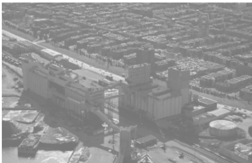
Silo #3 - Miron - Quais Laurier - dock Vrac Solide
