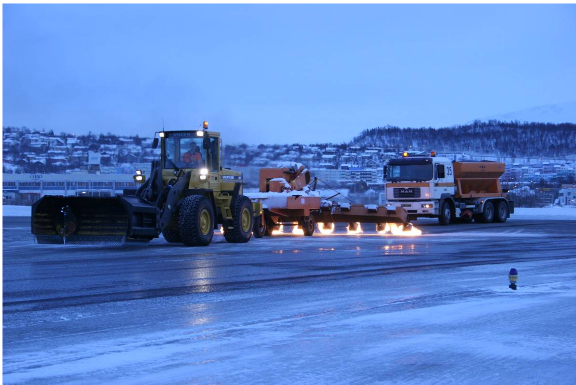
Figure 1. Traditional method of freeze bonding sand to pavement, practised at Norwegian airports. The iced pavement is heated by open flame burners prior to sanding.
