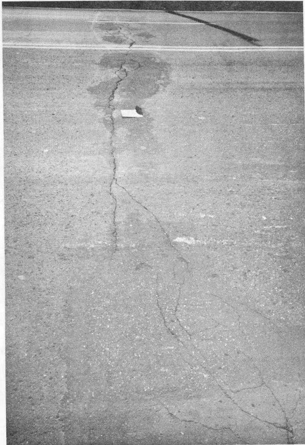
**Photo no3: FISSURE TRANSVERSALE**
